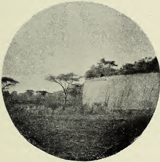
NORTH-EAST WALL OF TEMPLE, ZIMBABWE.
