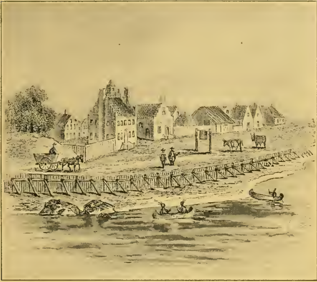
View of the "SCHOEINGE" or Sheet Piling on the East River Shore, near Coenties Slip, 1658
