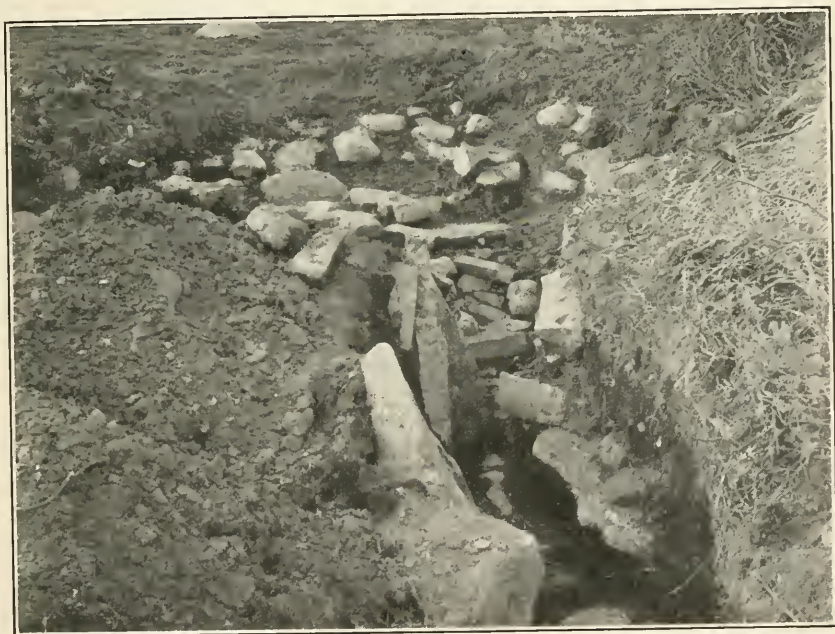
4. House of the old round type, seen from the entrance. Julianehaab district.
