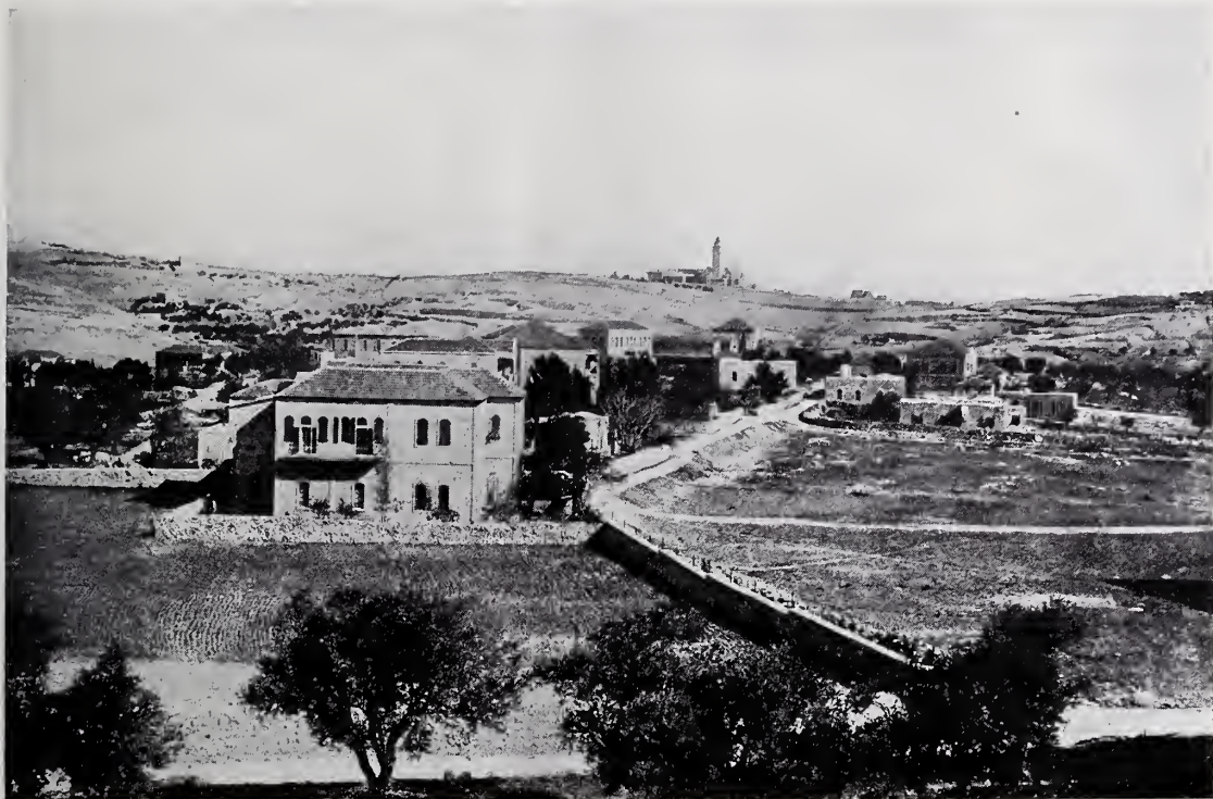
2. View of our property, looking East: The German Hospice on the Mount of Olives in the background
