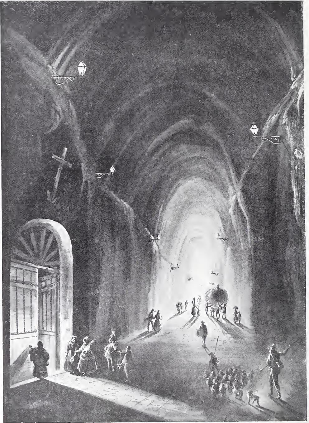
Fig 3. View of the Tunnel at Naples, about 1883.
