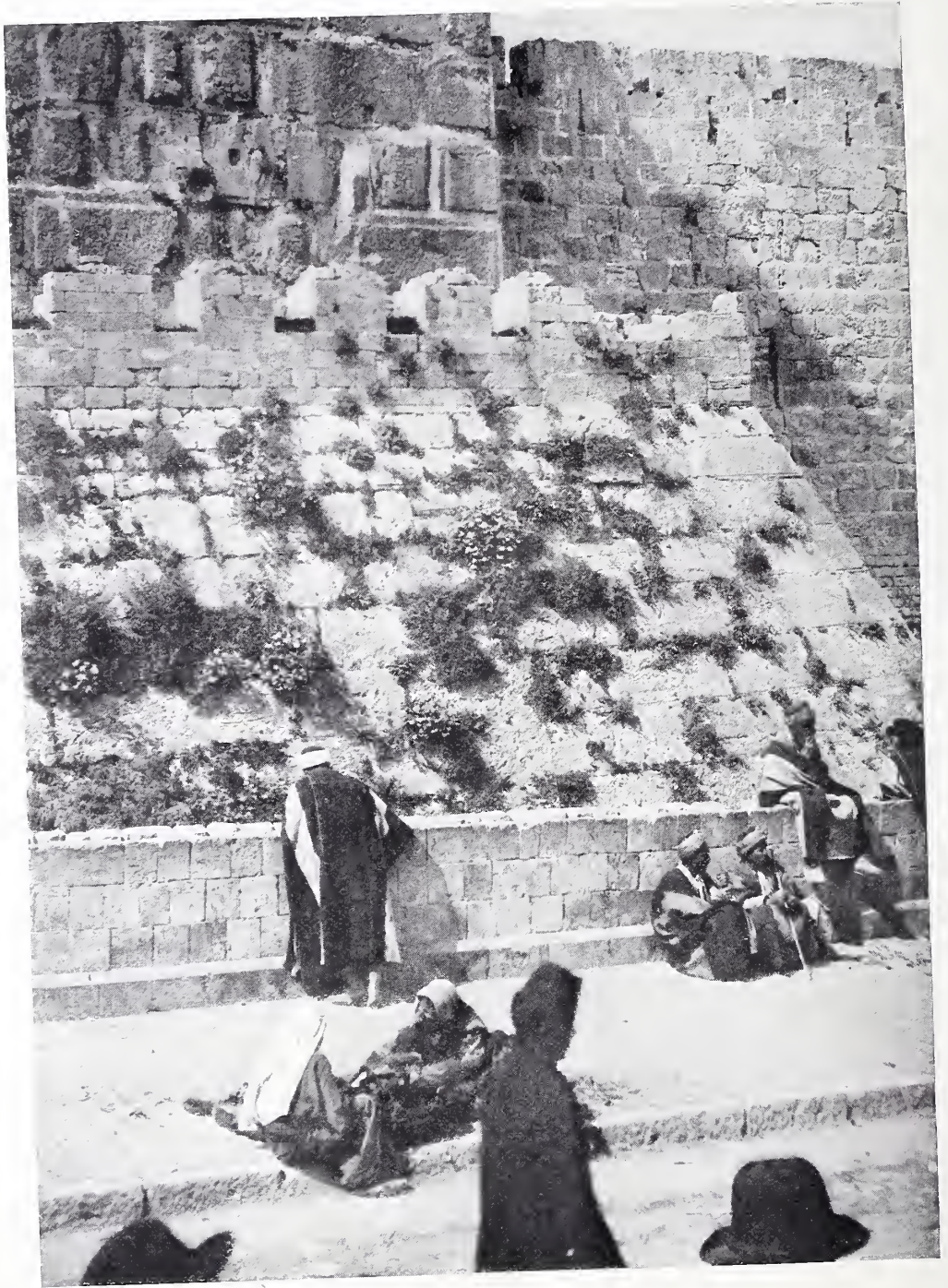
Ancient foundation of the northeast tower of the Citadel
