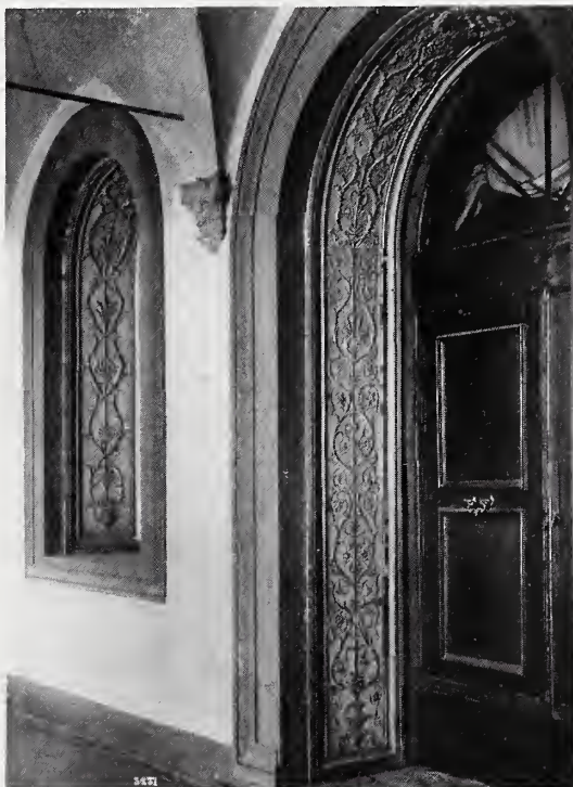
Brunelleschi. Detail of Doorway and Window in the Badia Fiesolana, Florence
