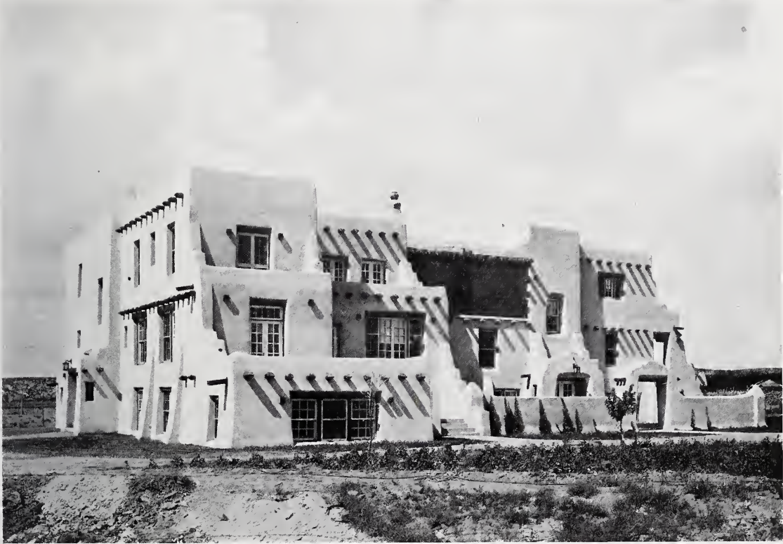
The Santa Fe School for Deaf Mutes. A formal expression of pueblo architecture
