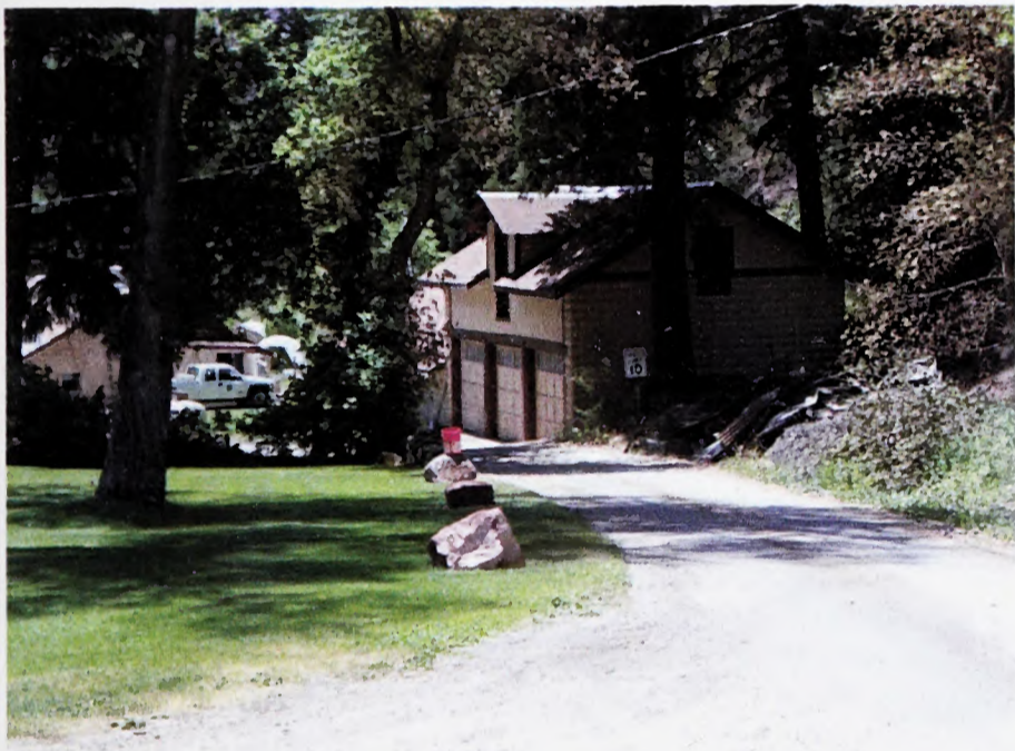
MITCHELL CREEK ROAD ABOVE HATCHERY – FLOOD FLOWS WILL BE CONVEYED DOWN THIS ROAD TO HATCHERY FACILITIES
