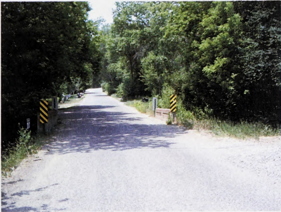
DONEGAN ROAD BRIDGE LOOKING WEST
