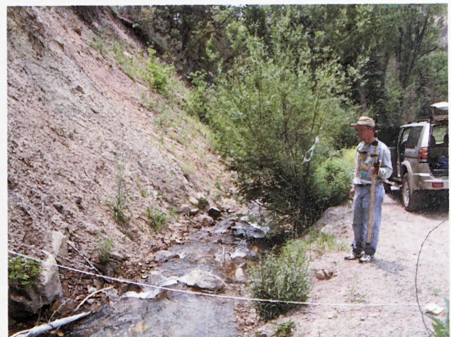
MITCHELL CREEK ROAD LOW POINT
