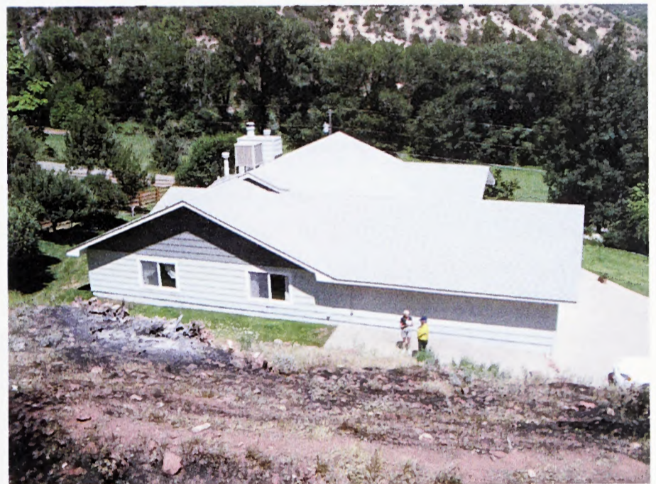
RESIDENCE ON WEST SIDE OF MITCHELL CREEK ROAD – DEBRIS FLOWS COULD DAMAGE THIS HOUSE.
