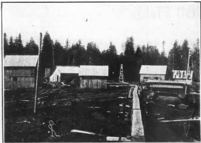
Oil field buildings of Chilcat Oil Co., at Katalla
