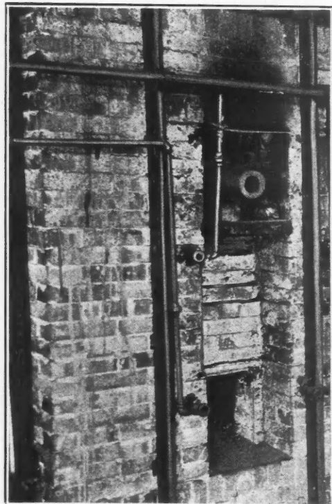
Fig. 2—Front view of Fiechtl furnace erected at Cherryvale, Kan.
