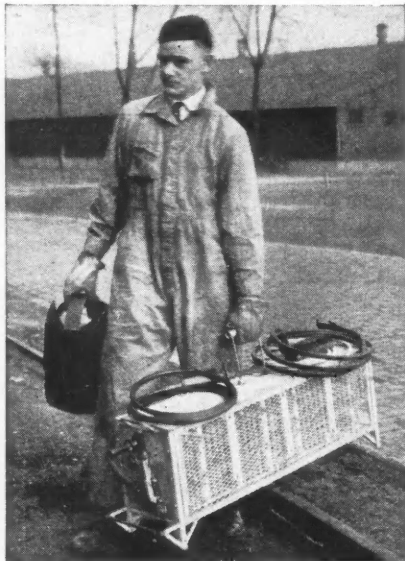
Machine for repair welding and rail bonding
