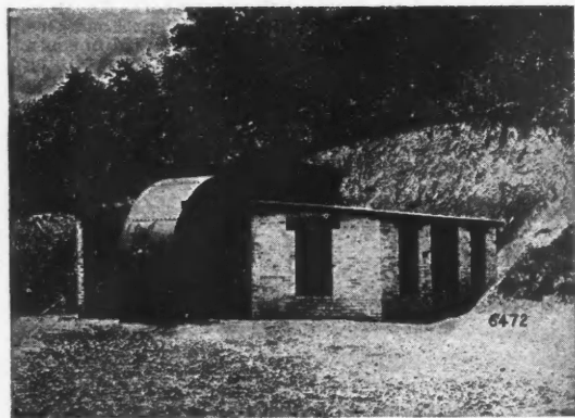
Double Inlet Reversible Fan. Capacity 200,000 cu.ft. at 3-in. water gauge.
