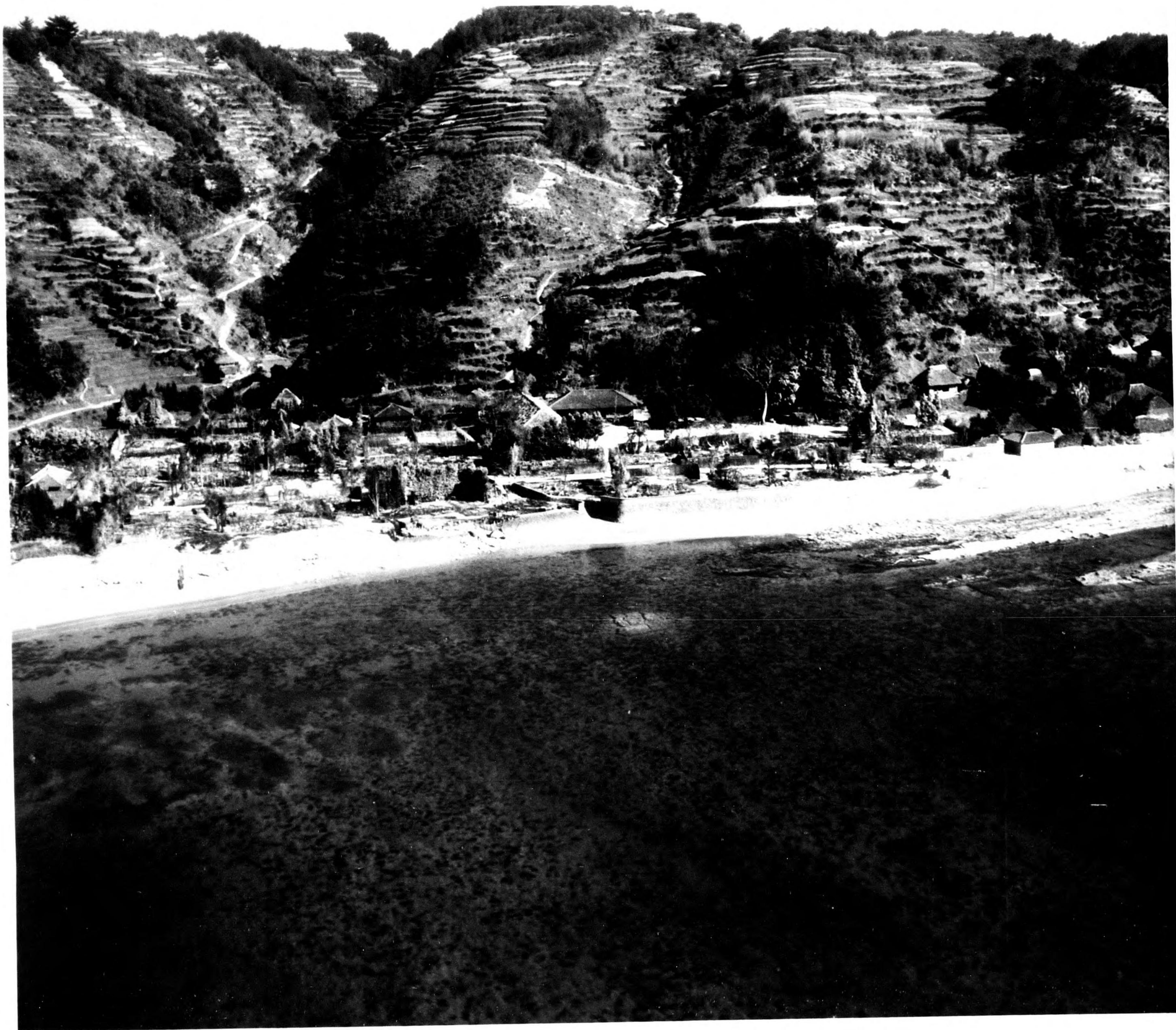
CVE 93-360 3 April 1945 OKINAWA SHIMA. View looking South showing sea wall at village of ANZA.
