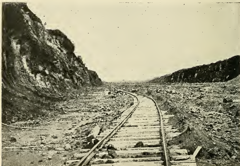
EXCAVATION FOR GATUN LOCKS COMPLETED.
