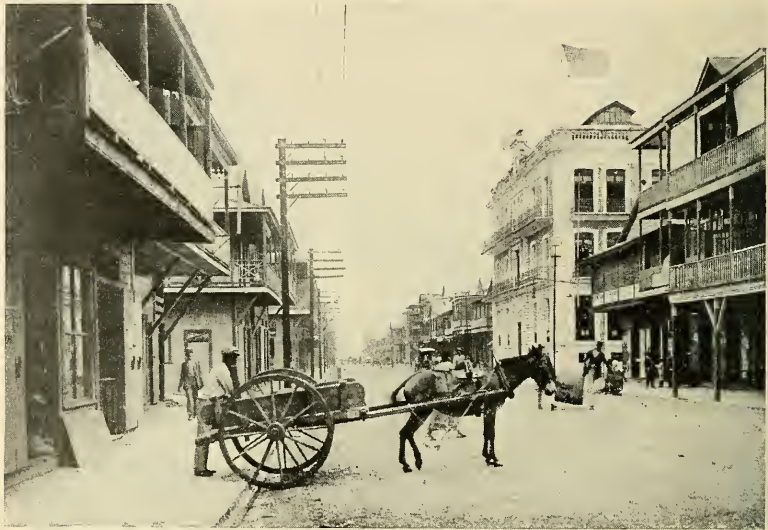
BOLIVAR STREET, COLON—AFTER AMERICANS HAD CLEANED AND PAVED IT.
