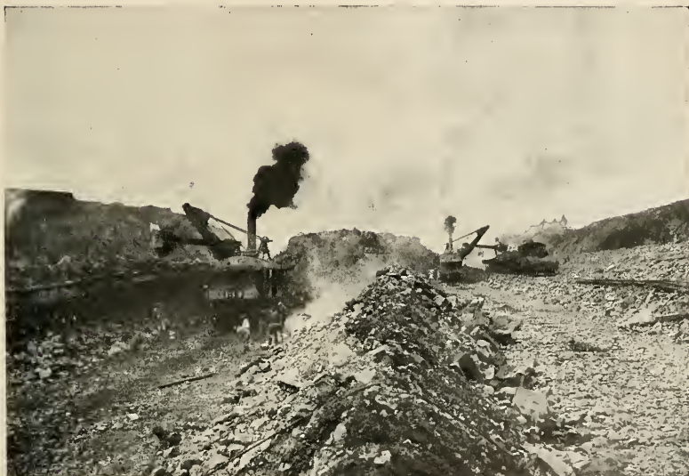
EXCAVATING FOR GATUN LOCKS.
