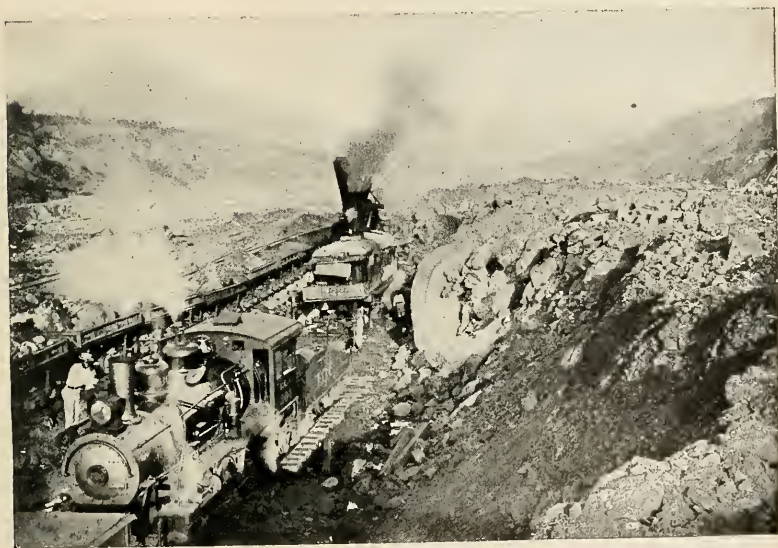
STEAM SHOVEL AT WORK ON THE SITE FOR THE PEDRO MIGUEL LOCKS.
