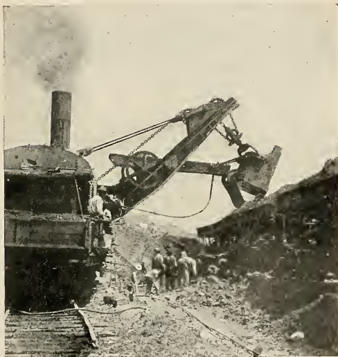
STEAM SHOVEL—SHOWING ARM AND DIPPER.
