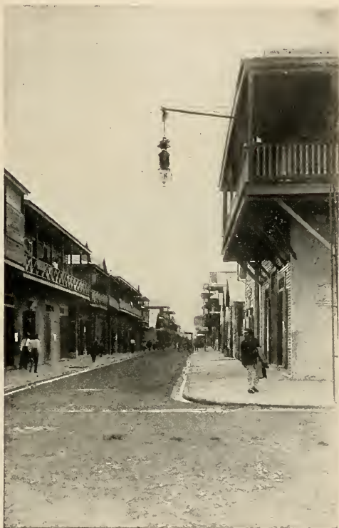
STREET IN COLON—PAVED AND CLEANED.
