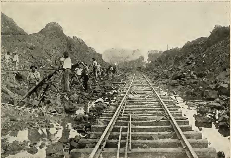
“MEN AT WORK DRILLING HOLES FOR THE CHARGES.”
