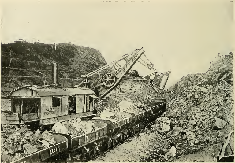
LOADING DIRT TRAIN BY STEAM SHOVEL.
