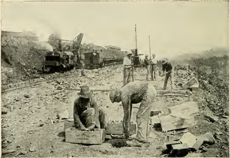
LOADING DRILL HOLES WITH DYNAMITE.
