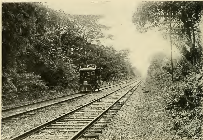
"NOW THE ROAD IS IN FIRST-CLASS CONDITION." Private car of Chairman of Isthmian Canal Commission.
