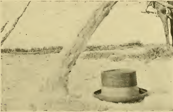
FIG. 18.—ALKALI EATING AWAY THE FENCE POSTS.
