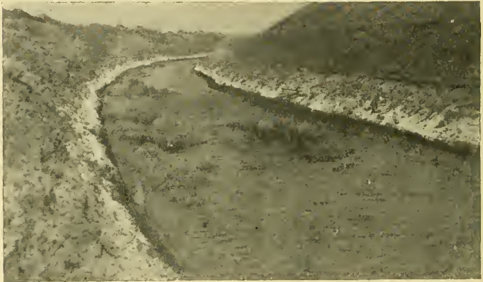
FIG. 22. — OPEN DITCH USED TO CARRY AWAY THE DRAINAGE WATER FROM A LARGE AREA. COVERED DRAINS EMPTY INTO THIS DITCH.
