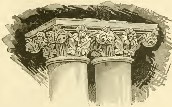
CAPS TO COLUMNS UNDER LADIES' GALLERY.
