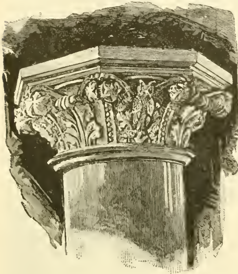
CAP OF LARGE COLUMN, ASSEMBLY ROOM.
