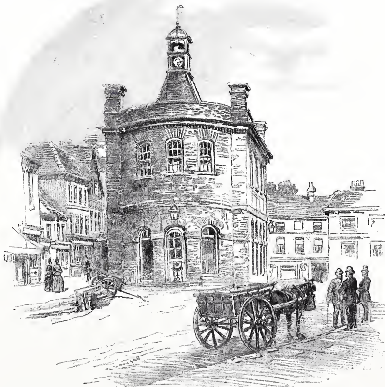
Town Hall, Reigate.
