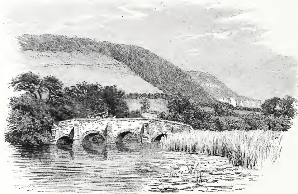
Bridge over the Mole.
