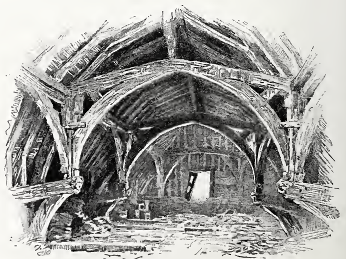
Roof of Strangers' Hall, Winchester.
