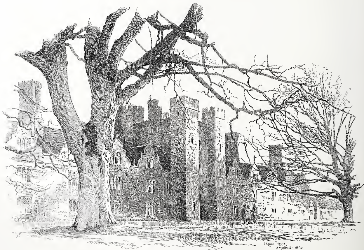
Fig. 1.—The Entrance Front.
