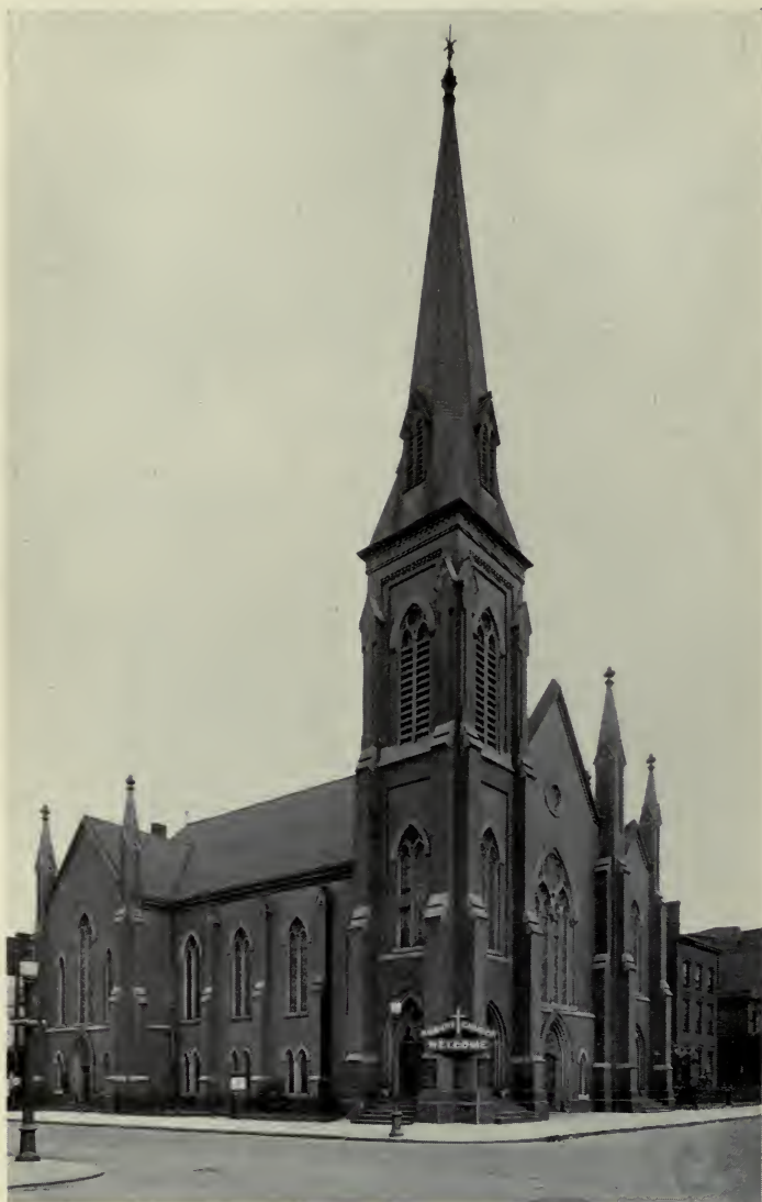
ASBURY M. E. CHURCH, PEARL AND CHIPPEWA STREETS. TORN DOWN, FOR ERECTION OF BUSINESS BLOCK, 1921-22.
