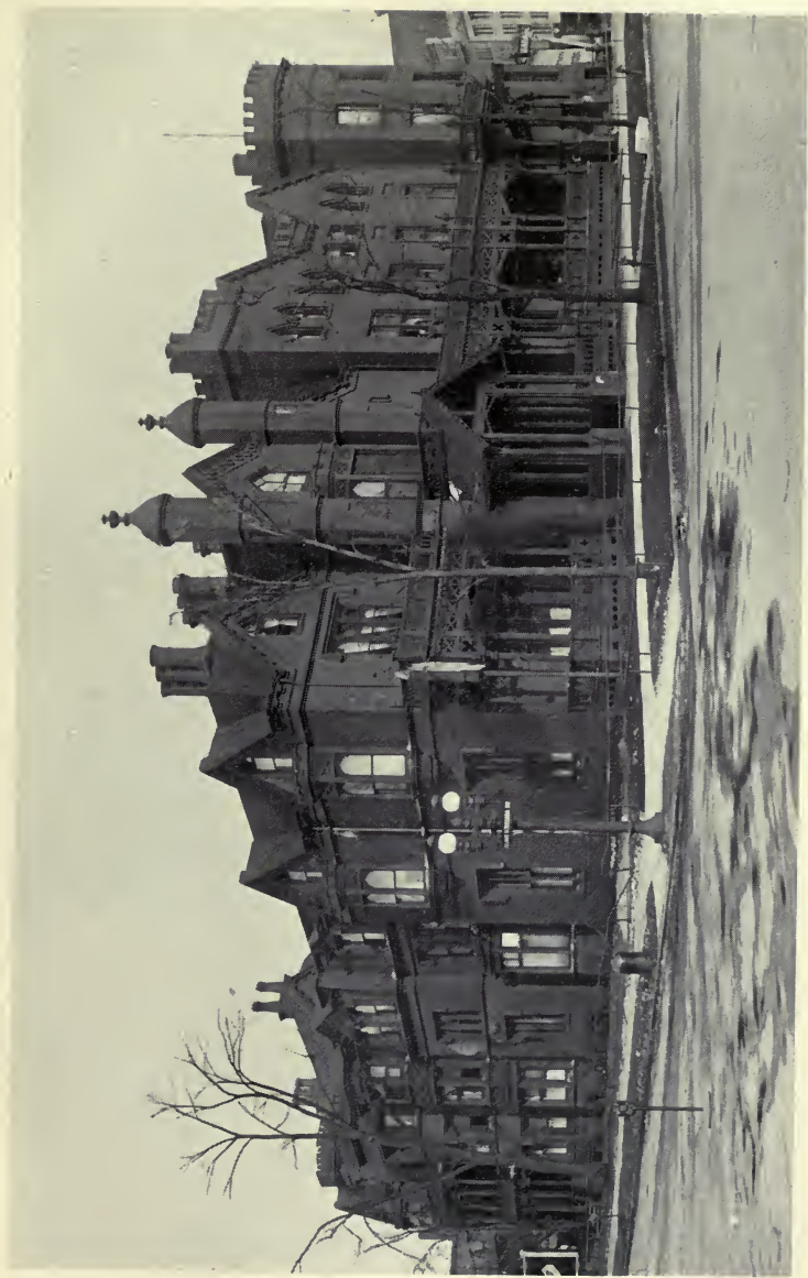
CASTLE INN, NIAGARA SQUARE, AS IT APPEARED JUST BEFORE BEING TORN DOWN, 1921.
