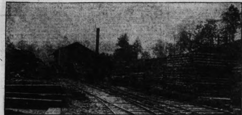
Rear End of Mill, Connecting Yard With Railway
