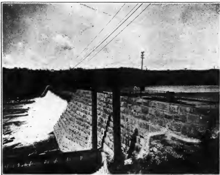
DAM AT PARAHYBA, TIETE RIVER, STATE OF SÃO PAULO, BRAZIL.
