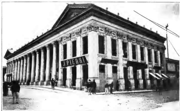
CITY HALL, QUEZALTENANGO, GUATEMALA.
