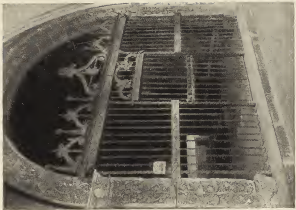
FIG. 99. REJA OF THE CAPILLA DE SANTA MAGDELENA. Cloisters of Tarragona Cathedral. Early XVI Century.
