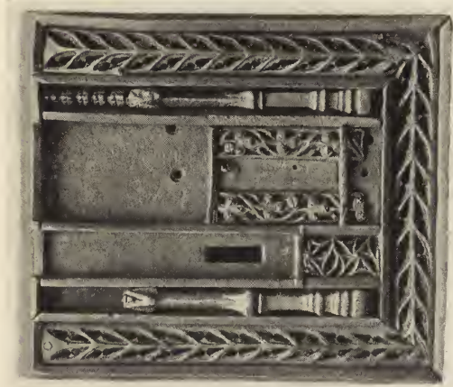
FIG. 73. CHEST LOCK WITH TYPICAL FIXING STAPLES.
