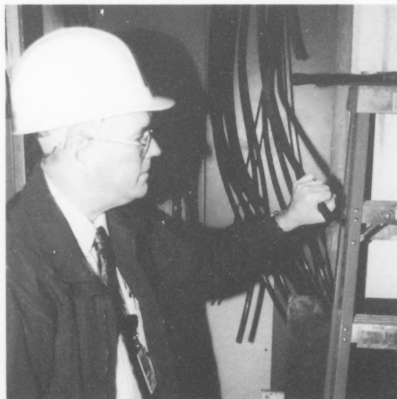
Project Officer John Helm inspects updated electrical service.
