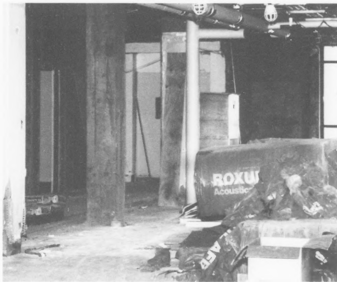
Contractors gut building to its concrete foundation before the rebuilding begins.
