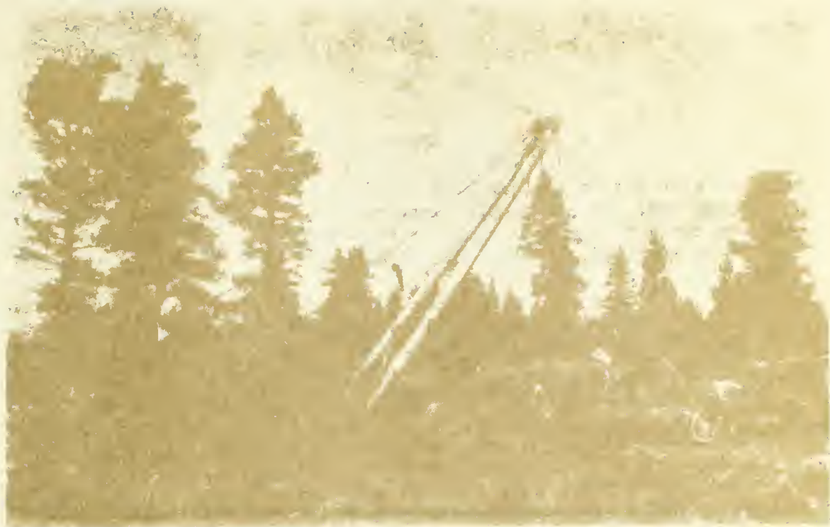
Figure 1. The Blacks Mountain portable log loader.
