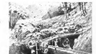
Edson's P. & M. Outfit conveying water from a distance to operate sluice. Capacity, 4,000 gallons per hour.
