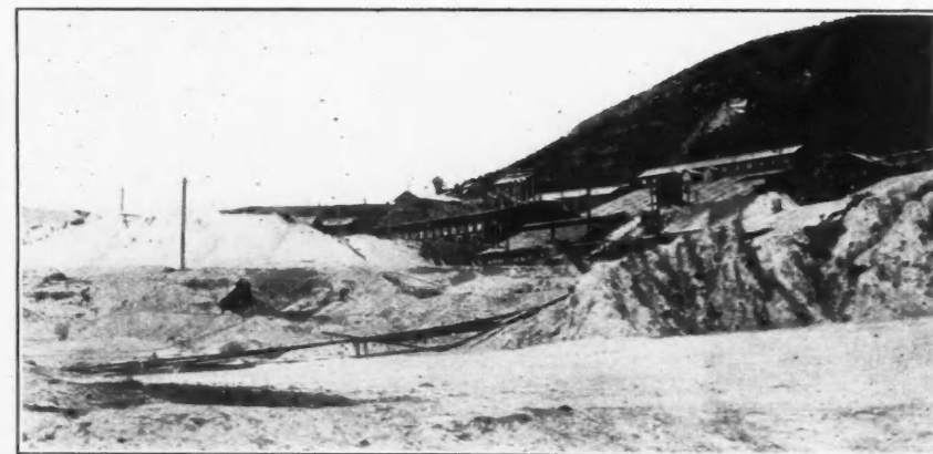
ESPERANZA MILL, SHOWING PORTION OF TAILINGS DUMPS
