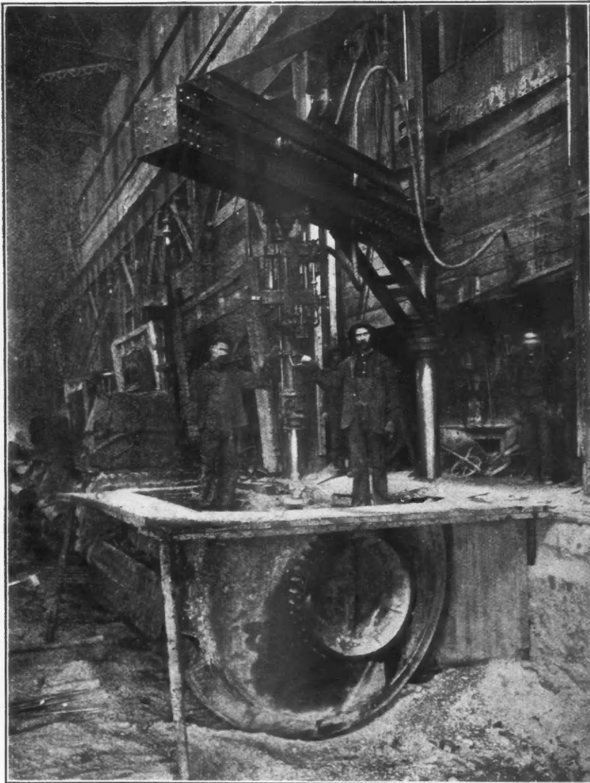
TAMPING CONVERTER LINING
