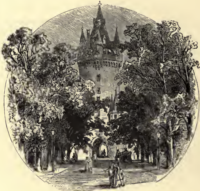
FRANKFURT-ON-THE-MAIN : ESCHENHEIM TOWER.
