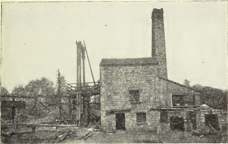
FIG. 10.—Engine House, Denby Grange Colliery, showing gin and capstan on the left.
