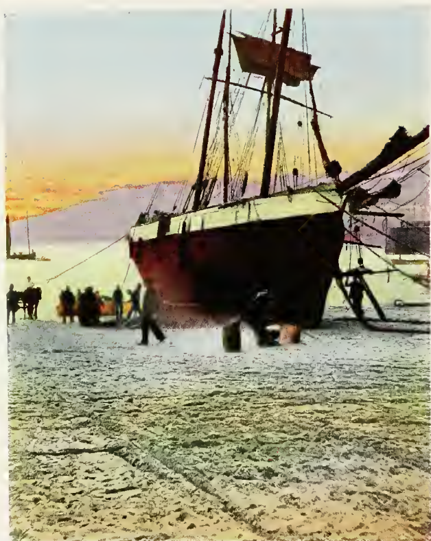
ASHORE FOR REPAIRS — ST. IVES.
