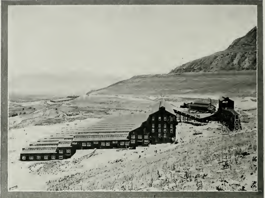
Concentrator Plant, Boston-Consolidated Mining Company, Garfield, Utah
