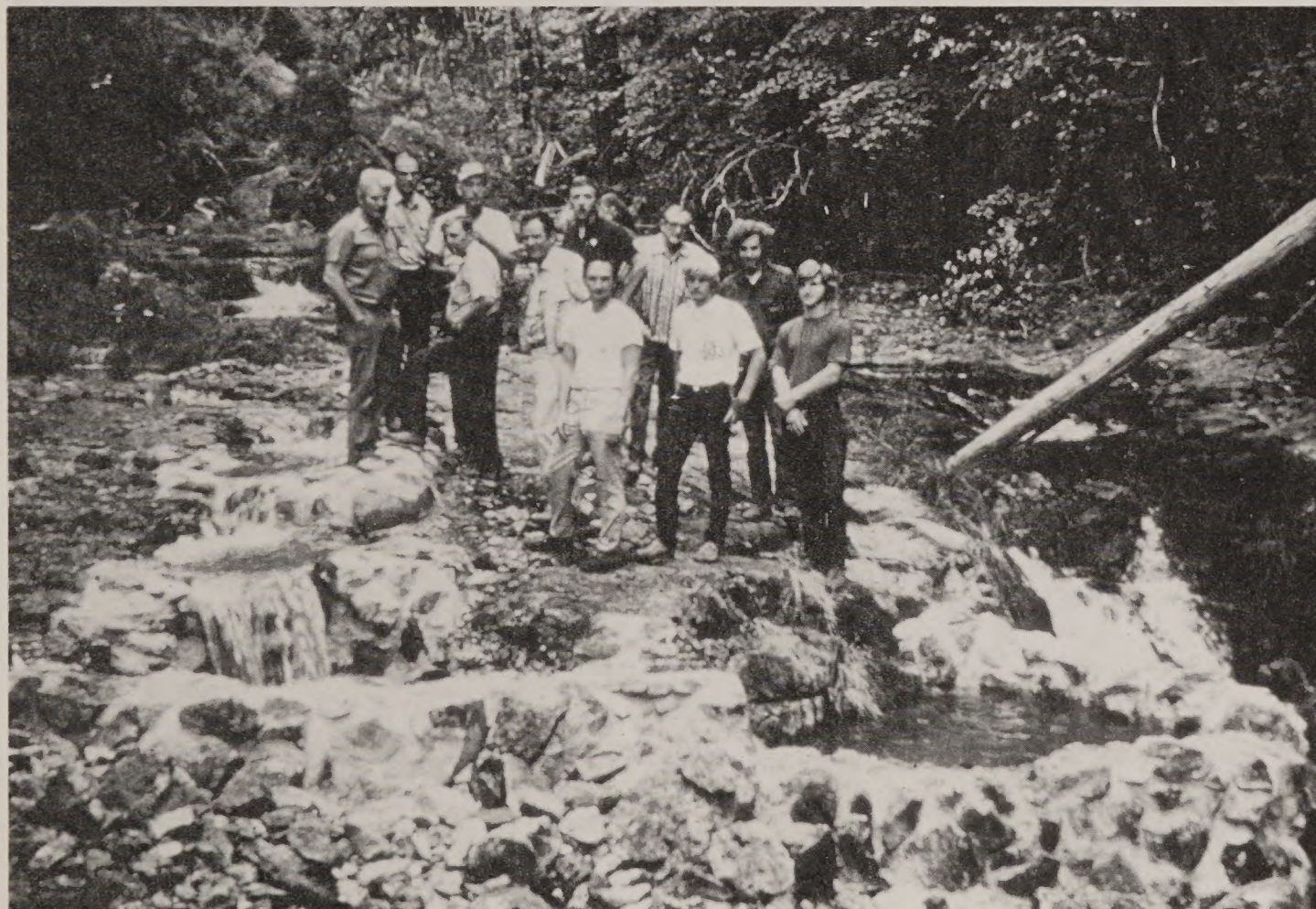
7. Volunteers stand by a series of jump pools they helped construct which will allow adult salmon to negotiate waterfalls and reach spawning areas upstream.
