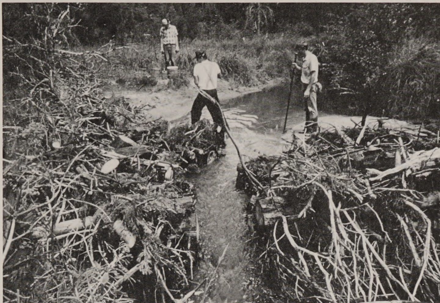
6. Bureau personnel remove woody debris that blocks upstream migration of anadromous fish.
