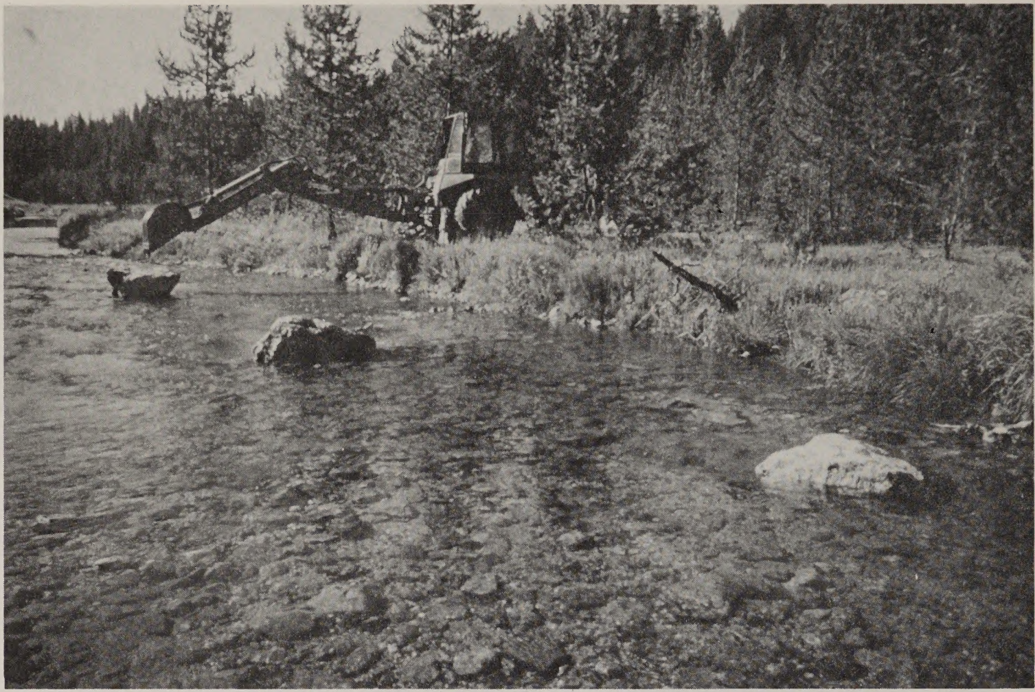
12. Large boulders are individually placed by heavy equipment to create pool habitats of young and adult fish.
