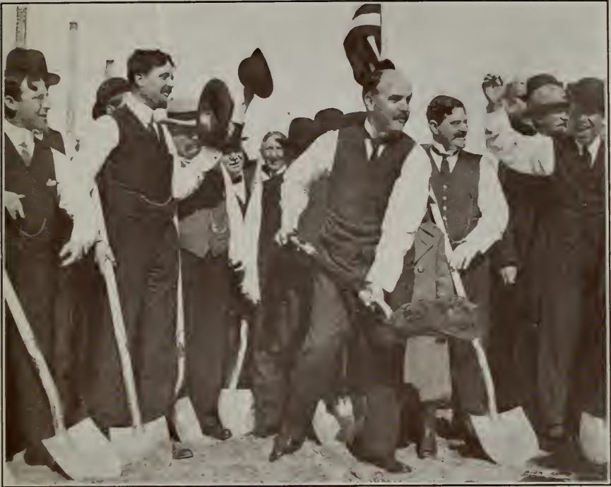
MAYOR ROLPH BREAKING GROUND FOR NEW CITY HALL
