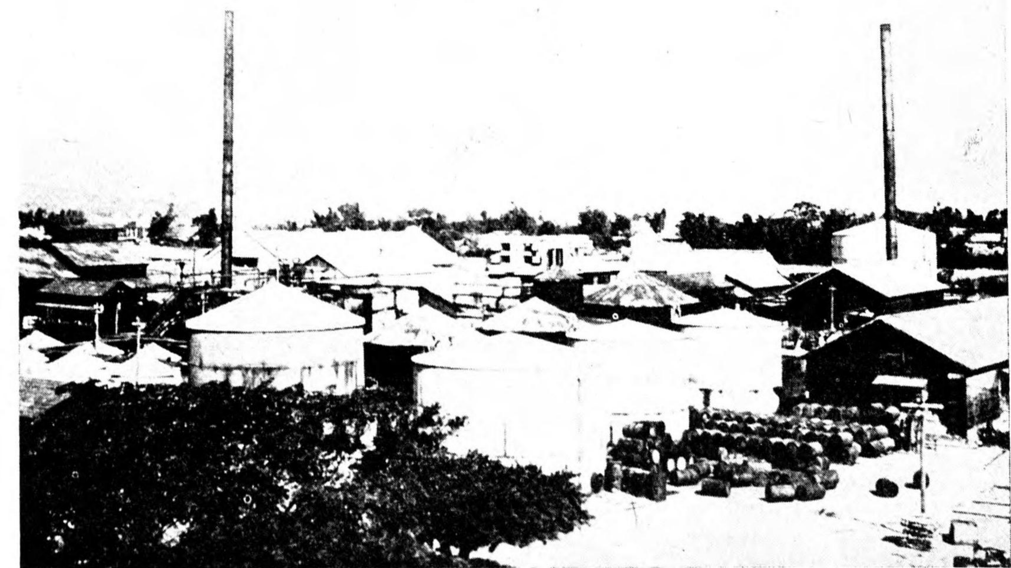
10. Oil storage tanks at Byoritsu.
