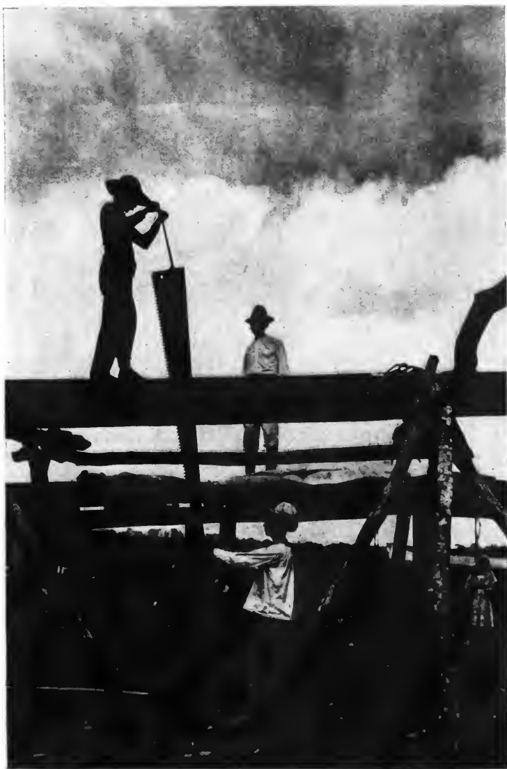
SAWING THE LOG INTO LUMBER.
