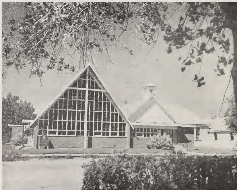
Coaldale United Church, with its high gable, combines modern and traditional design
