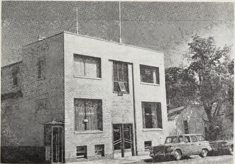
Town office, library, police office and health unit are located in this administration building
