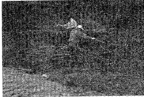
Unemployed fishermen build willow wall field overgrazed, eroding stream bank.
