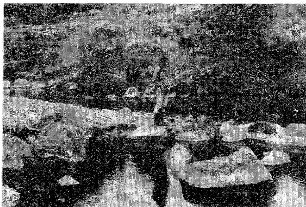
AFTER Installation of boulder weirs to collect spawning gravel and to create deeper pools. Barbs installed to deflect flow toward center of stream.
