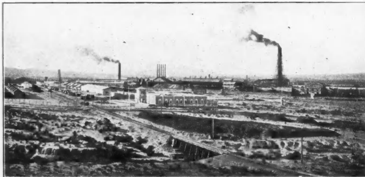
SMELTER OF THE COMPANIA MINERA DE PINOLES, AT MAPIMI, DURANGO, MEXICO, WHERE TWO NO. 1 WHITE BRIQUETTING PRESSES ARE BEING ERECTED.
