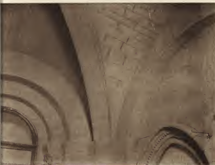
FIG. 20. St. - Victor, Marseille. Vault of Porch.
