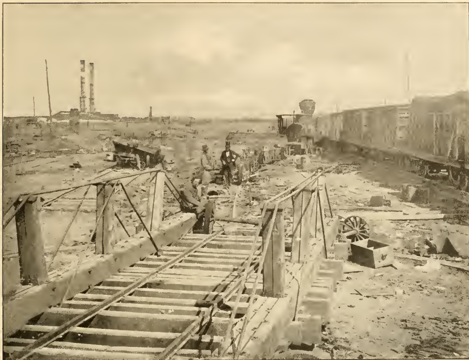
DESTRUCTION OF RAILROAD AT MANASSAS.
