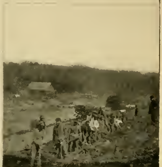
U.S. Engineers Constructing road on South bank of North Anna River.
