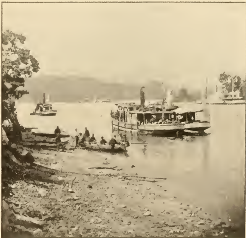
TRANSPORT AND MONITOR ON JAMES RIVER.
