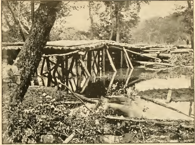
BRIDGE ACROSS CHICKAHOMINY RIVER, BUILT BY 15TH NEW YORK ENGINEERS.
