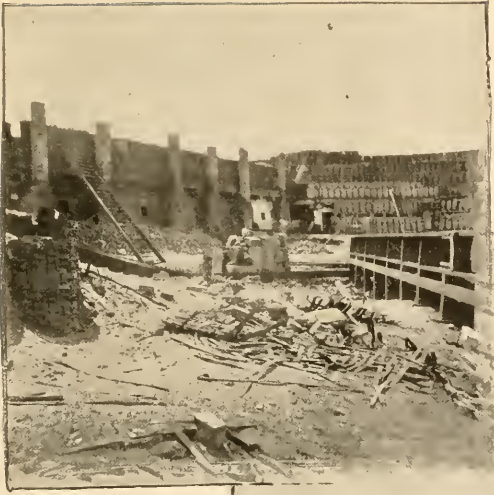
INTERIOR VIEW, SHOWING HOW WALLS WERE STRENGTHENED.
