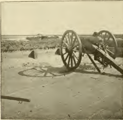
VIEW OF PARAPET, FORT SUMTER.
