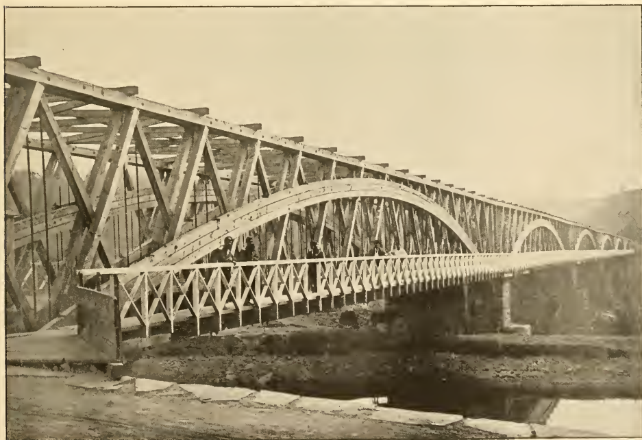
CHAIN BRIDGE, POTOMAC RIVER.
