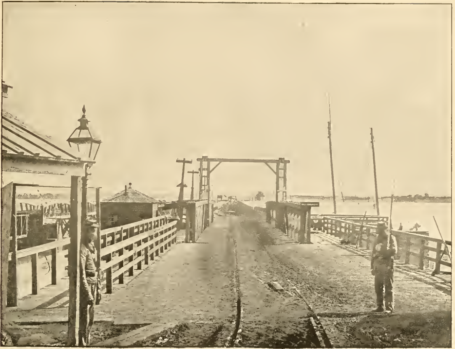
LONG BRIDGE, WASHINGTON.
