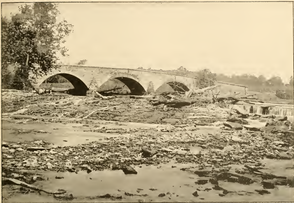
ANTIETAM BRIDGE, LOOKING UP STREAM.
