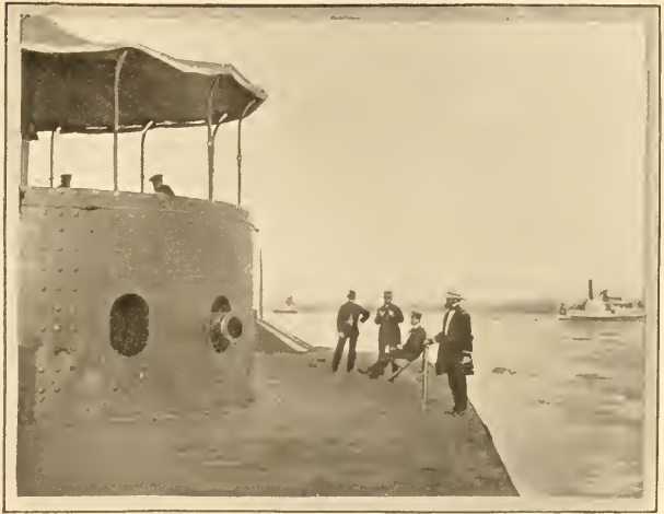
TURRET AND PART OF DECK OF ORIGINAL MONITOR, SHOWING DENTS MADE BY LOUNTED SHOT FROM THE GUNS OF THE "MERRIMAC."
