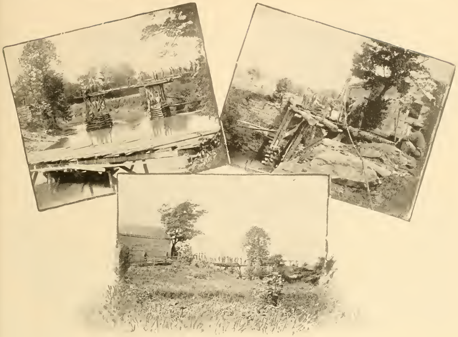
TROOPS BUILDING BRIDGE ACROSS NORTH FORK RAPPAHANNOCK RIVER, NEAR FAUQUIER SULPHUR SPRINGS.
