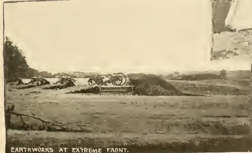
EARTHWORKS AT EXTREME FRONT.
