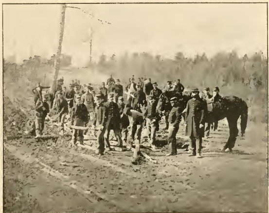
ENGINEER CORPS MAKING CORDUROY ROADS.
