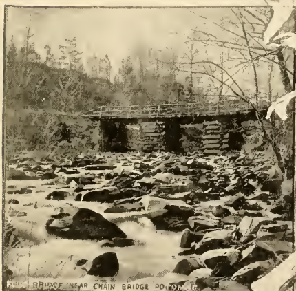
BRIDGE NEAR CHAIN BRIDGE POTOMAC.
