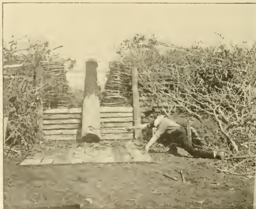
CONFEDERATE FORTIFICATION AT CENTREVILLE, AFTER EVACUATION, MARCH, 1862.
