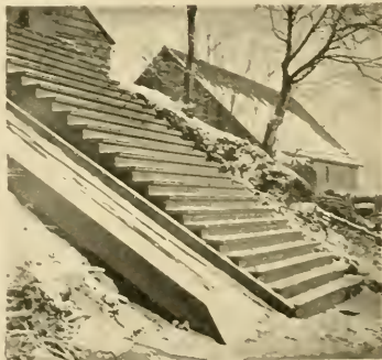
Stairways Side of Commissary Building.
