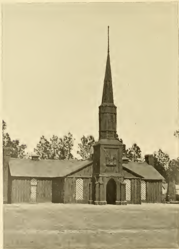
CHURCH BUILT BY THE ENGINEERS
