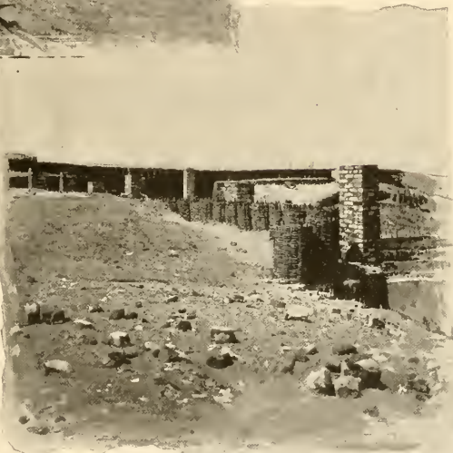
INTERIOR VIEW ON PARAPET.
