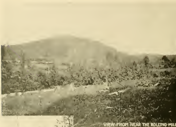
VIEW FROM NEAR THE ROLLING MILL
