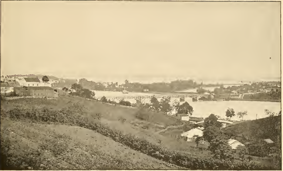
AQUEDUCT BRIDGE, POTOMAC RIVER.
