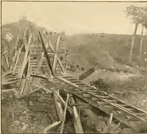
TRACK AND BRIDGE DESTROYED ON VIRGINIA CENTRAL RAILWAY.
