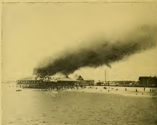
THE SOUTH END PAVILION, FORMERLY "LILLAGORE'S," WAS TOTALLY DESTROYED BY FIRE ON APRIL 21ST, 1915
