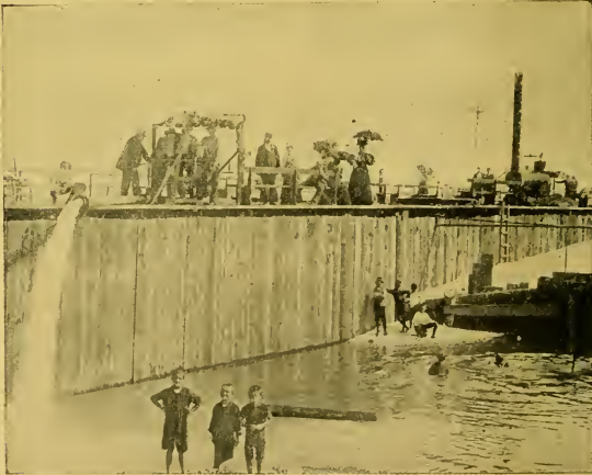
STARTING THE SAND PUMP
