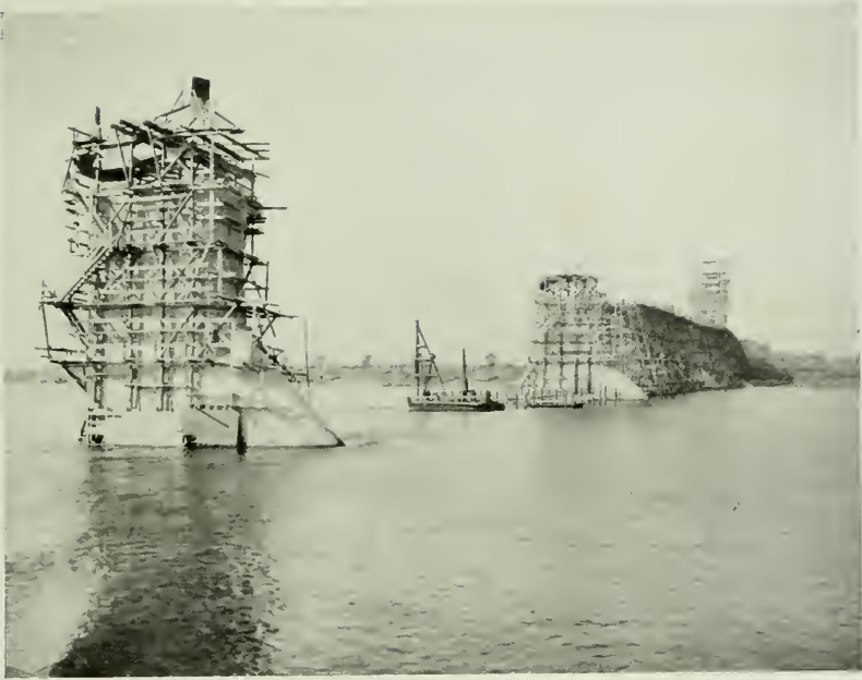
THE RAILWAY BRIDGE ACROSS THE SEVA, AT ALEXEYEVSK (OCT. 13)
