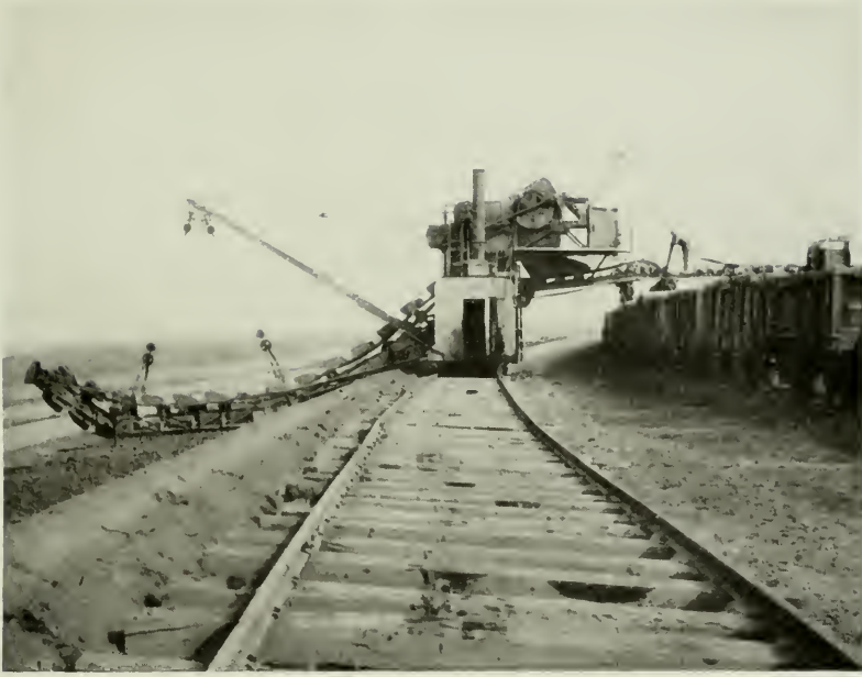
THE EXCAVATOR AT WORK, DIGGING A CHANNEL FOR DRAINAGE (OCT. 7)
