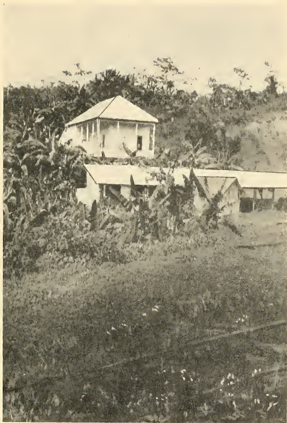
ALONG PANAMA RAILROAD
