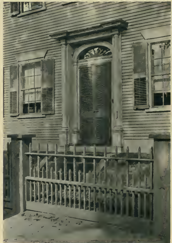
DOORWAY, CORNER OF UNION AND HIGH STREETS, BRISTOL, RHODE ISLAND
