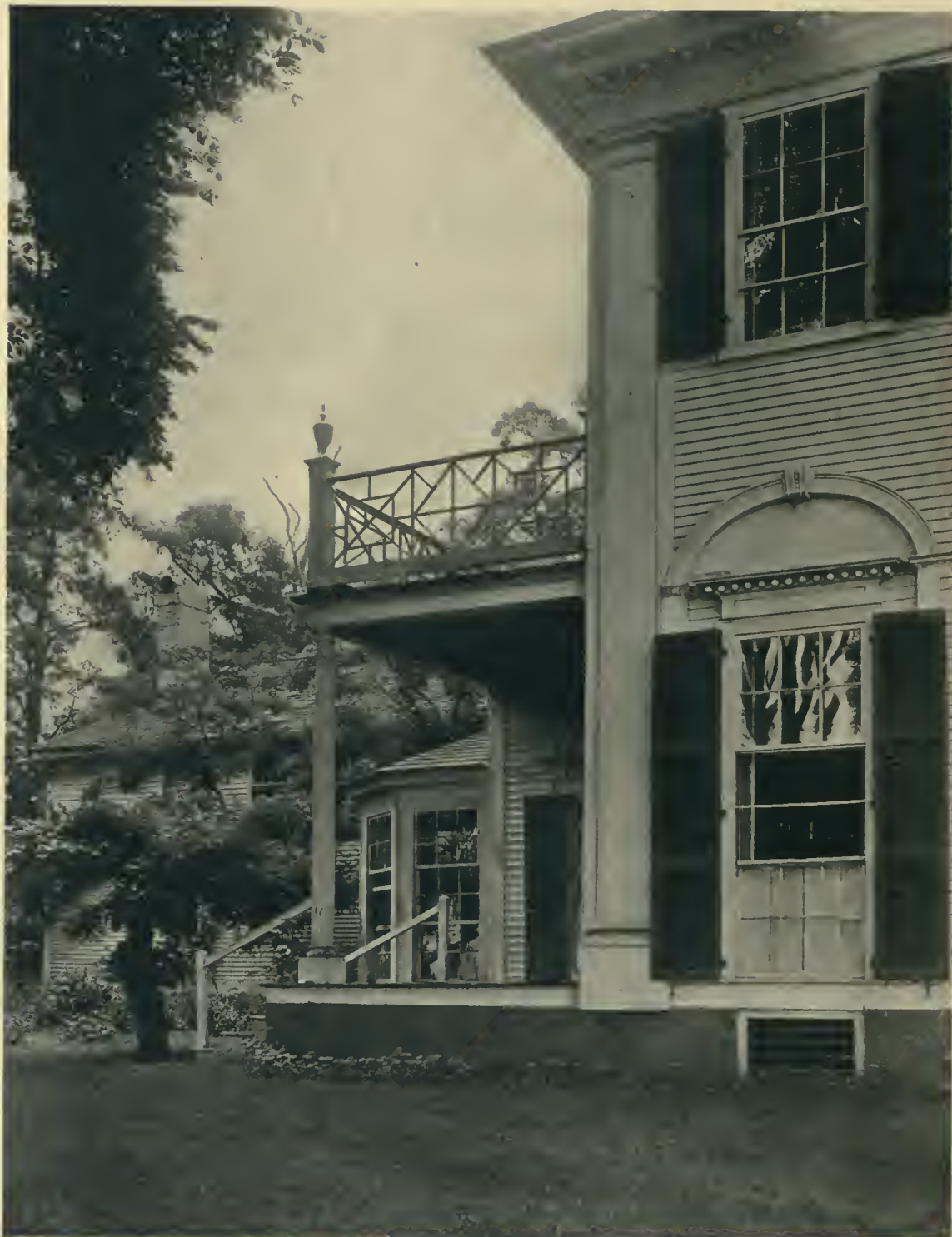
THE DE WOLF-MYDDLETON HOUSE, BRISTOL, RHODE ISLAND. Detail of East Front. RUSSELL WARREN, ARCHITECT.
