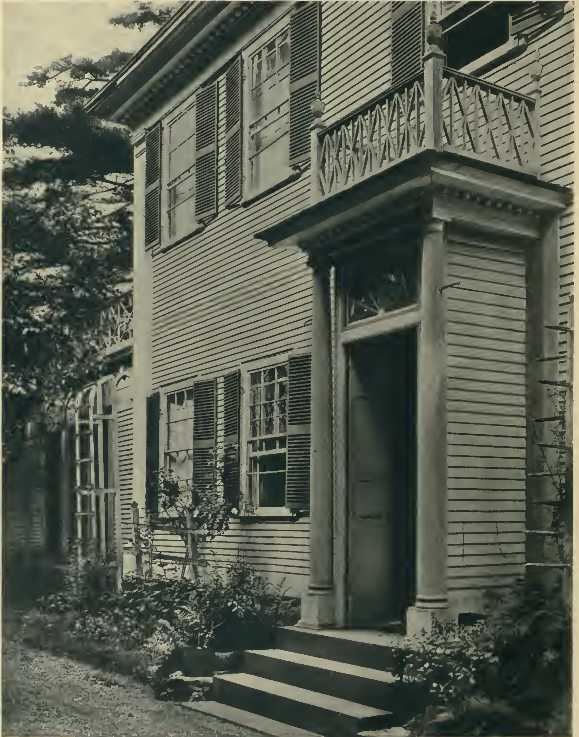
THE DE WOLF-MYDDLETON HOUSE, BRISTOL, RHODE ISLAND. Detail of West Front and Entrance. RUSSELL WARREN, ARCHITECT.
