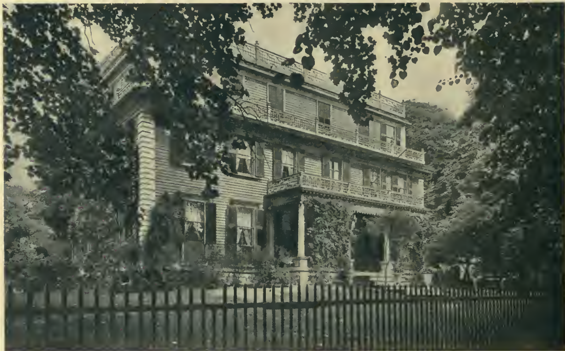
THE NORRIS HOUSE, BRISTOL, RHODE ISLAND. Date about 1810. Celebrated for its exaggerated amplification of the Rhode Island cupola motif until it covers, practically, the entire roof of the building.
