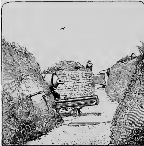
INTERIOR OF FORT PUTNAM, FORMERLY THE CONFEDERATE BATTERY GREGG, CUMMING'S POINT, S. C. FROM A PHOTOGRAPH.
