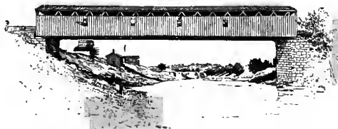
BRIDGE AT FRANKLIN OVER THE HARPETH RIVER, LOOKING UP-STREAM.
