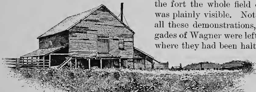
FRONT VIEW OF THE GIN-HOUSE.
