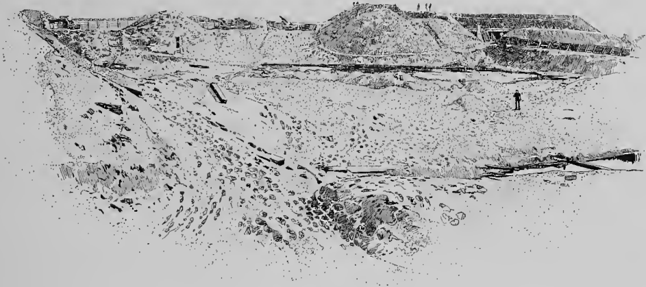
INTERIOR VIEW OF THE NORTH-EAST ANGLE. FROM A PHOTOGRAPH.
