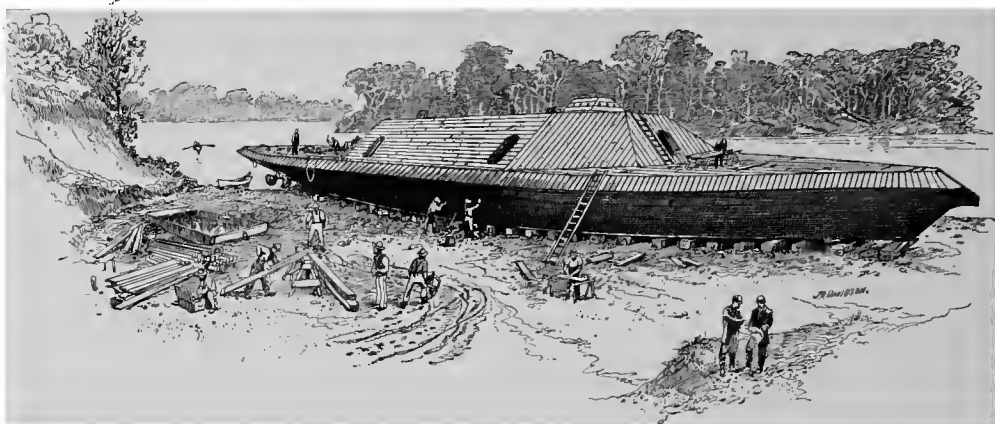
BUILDING THE "ALBEMARLE" AT EDWARDS'S FERRY.
