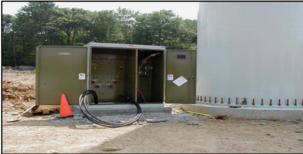
Figure 35. Typical pad-mounted transformer under construction.
