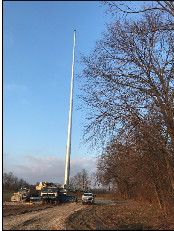
Figure 16. Typical monopole meteorological tower.
