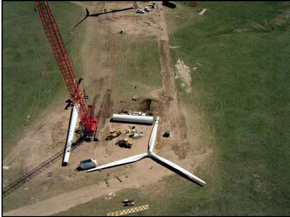
Figure 27. Aerial view of preparations to erect a wind turbine tower.
