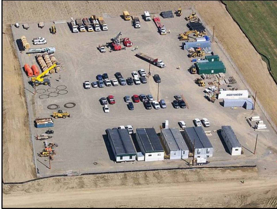
Figure 17. Typical storage/staging/laydown area during construction.
