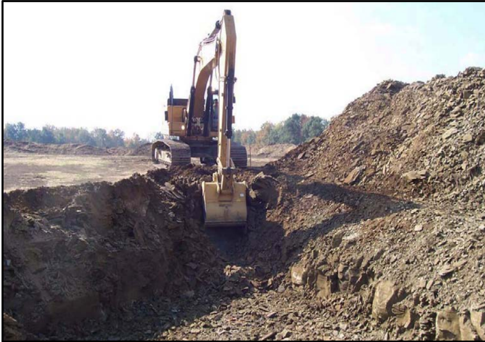
Figure 22. Excavating foundation hole.
