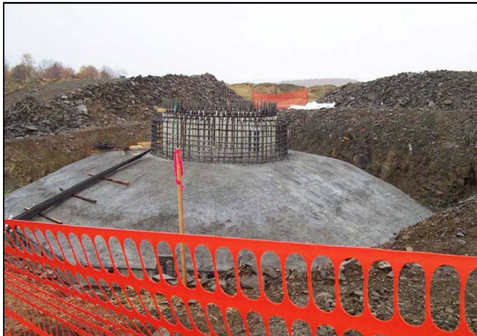
Figure 25. Typical spread-footing foundation.
