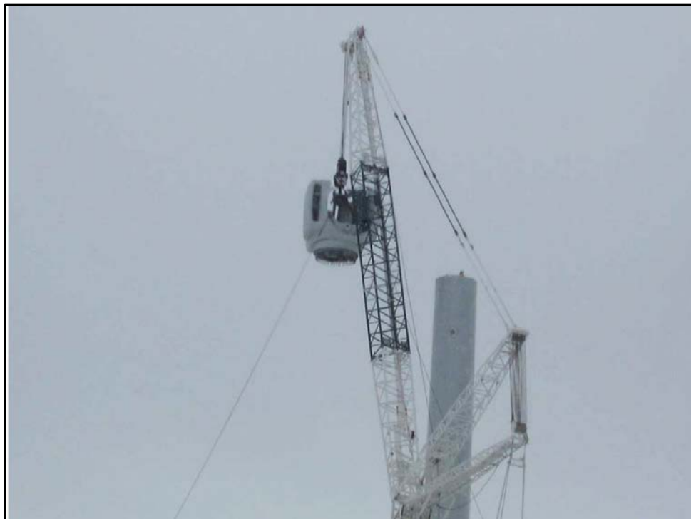
Figure 28. Wind turbine nacelle installation.
