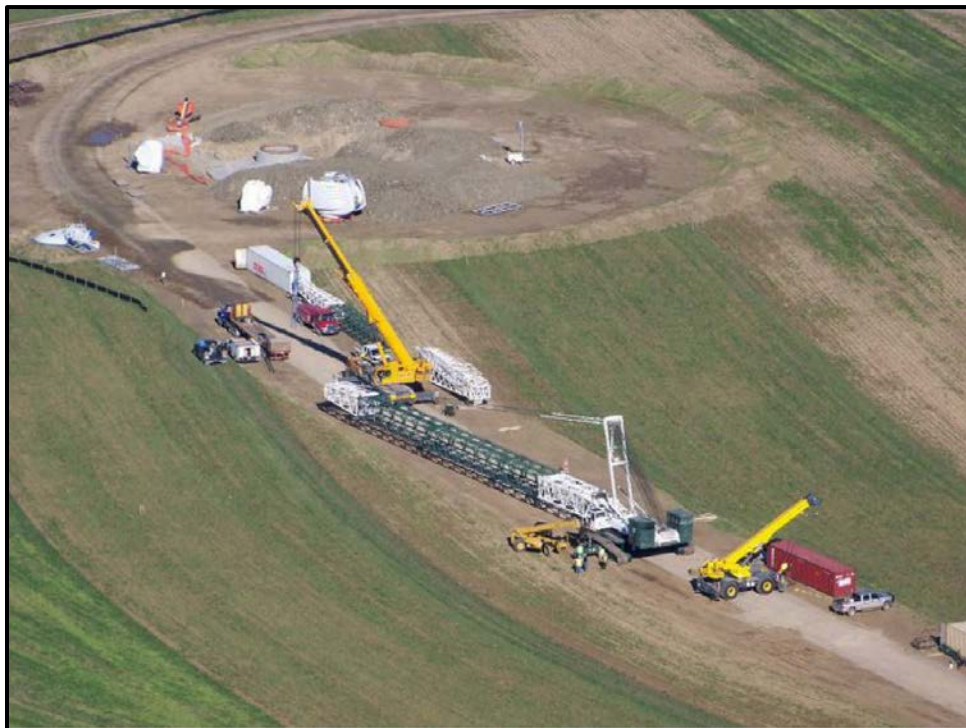
Figure 26. Turbine erection.
