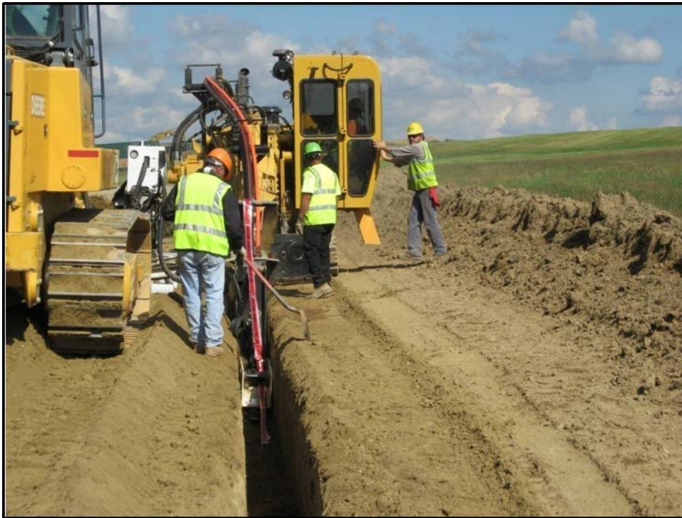
Figure 33. Typical underground collector cable trench.
