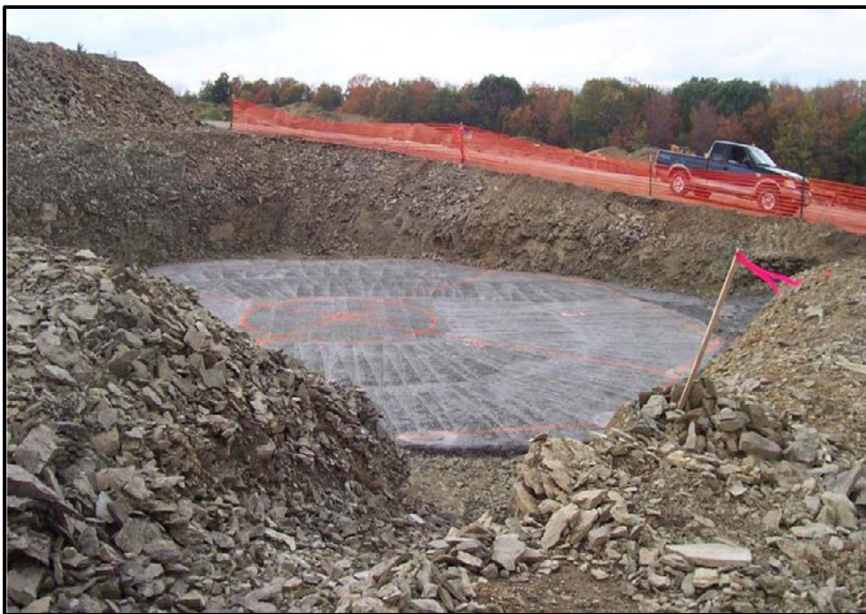
Figure 23. Excavated foundation area.
