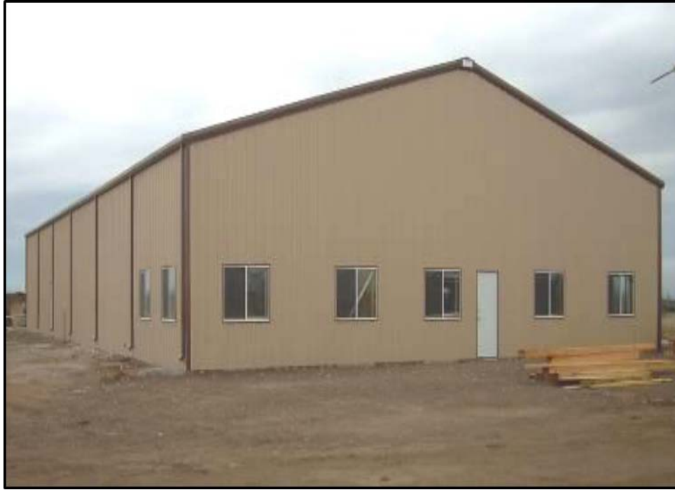
Figure 15. Typical O&M building.
