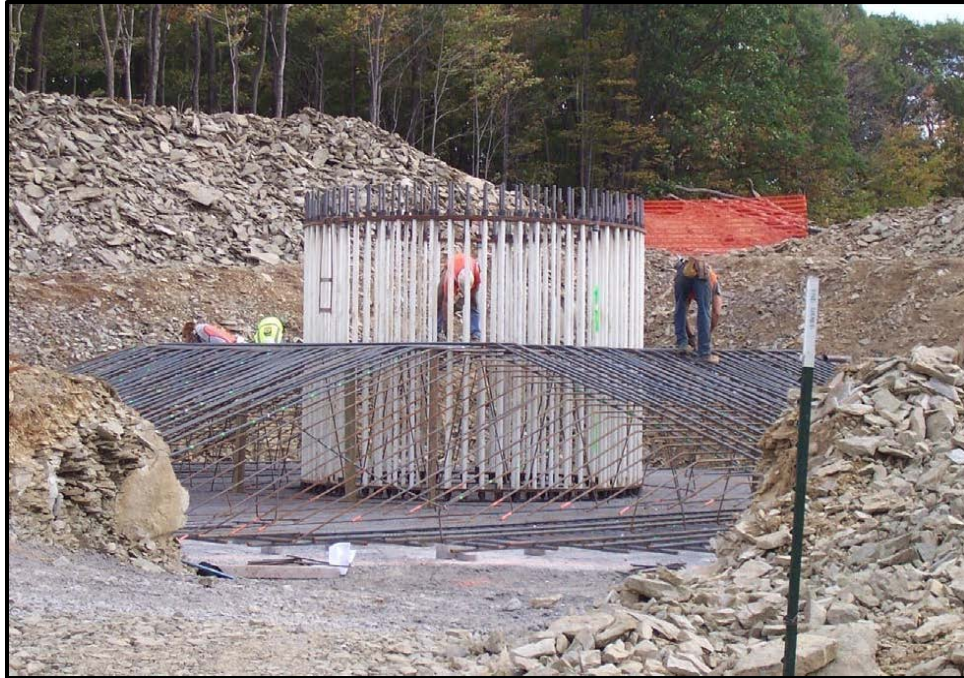
Figure 24. Foundation rebar and bolt cage.
