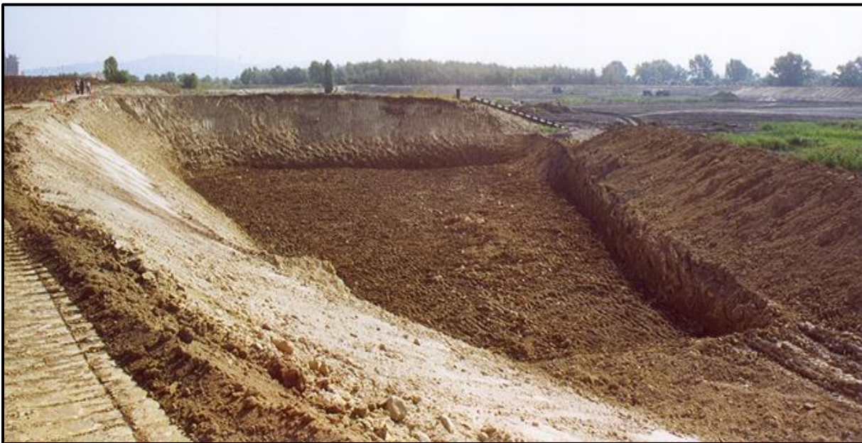
Figure 19. Typical borrow pit.
