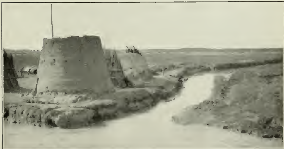
FIG. 3.—INTAKE OF IRRIGATION CANAL ABOVE BASSORAH.
