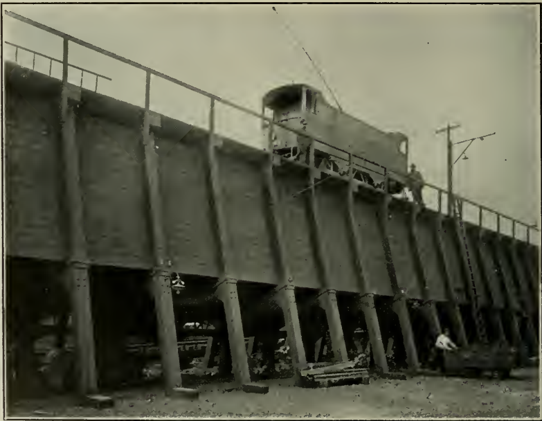
COAL POCKET AT AN INLAND STATION.
