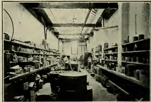
THE PAINT-MIXING ROOM.
