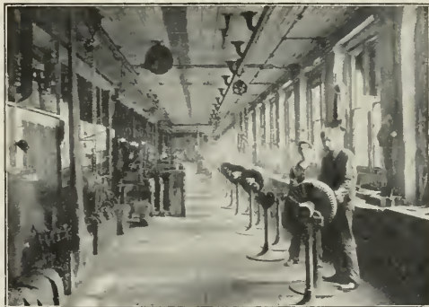
ARMATURE, COMMUTATOR, AND COIL REPAIR SHOP.
