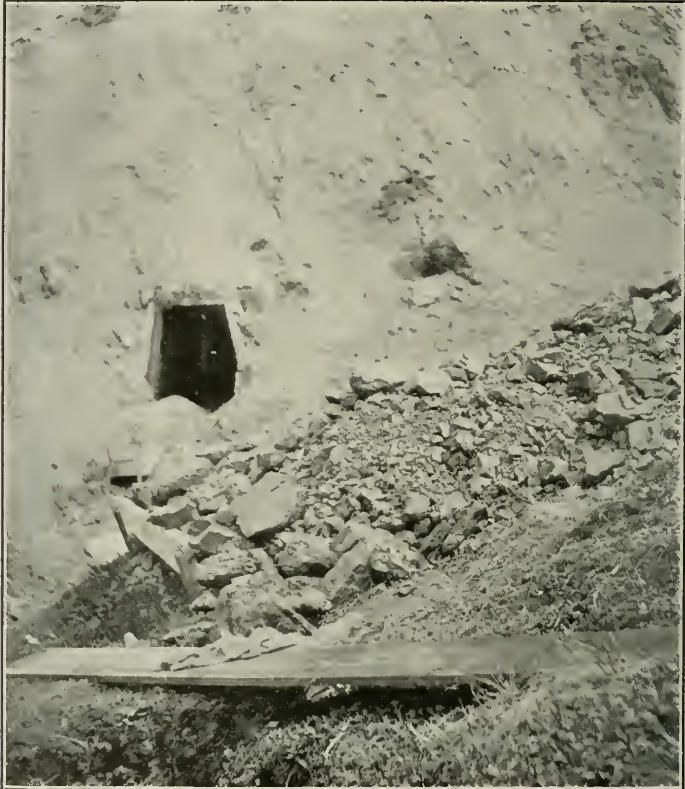
RECENT TUNNEL INTO NEWLY DISCOVERED COAL SEAM ON HERENDEEN BAY Lat. 55^{\circ} 45' N. , long. 160^{\circ} 40' . At the end of tunnel, seam is 53 inches thick. Pile of coal in foreground.
