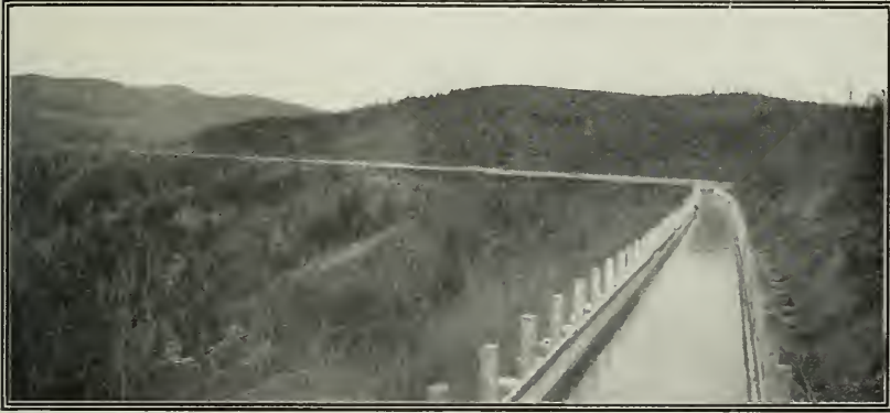
FORTY THIRD COMPANY'S DITCH, KILDARE GULCH, OMINECA.
