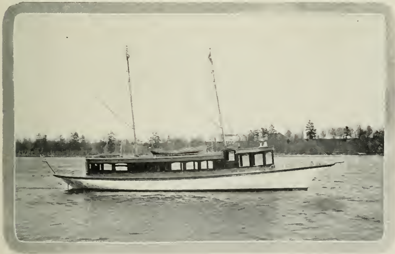
YACHT 53 BY 10 FEET, 18-HORSE-POWER THREE-CYLINDER SELF-STARTING AND REVERSING ENGINE.
