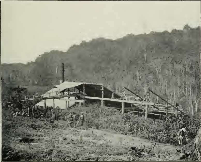
THE TAMSU MILL, LOOKING FROM THE TOP OF THE RIDGE.
