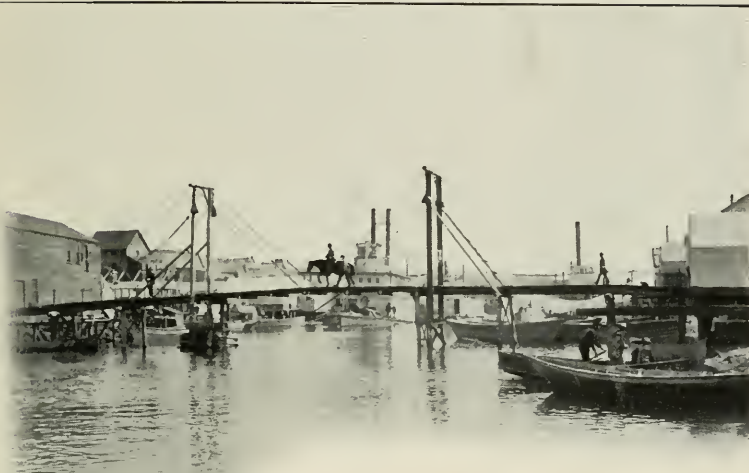
BRIDGE ON SNAKE RIVER, NOME CITY.
