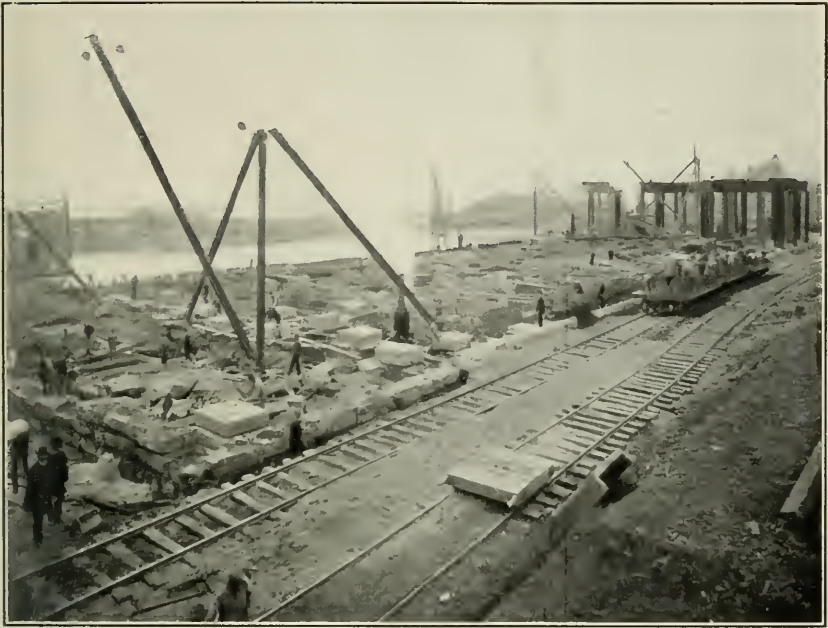
SETTING MASONRY PEDESTALS FOR THE FOUNDATIONS OF A GREAT TANK-BIN ELEVATOR.
