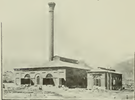
POWER HOUSE, CANYON CITY, COLORADO.
