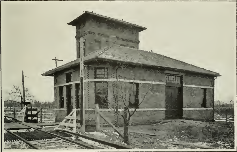
SUB-STATION, G. R., G. H. & M. RY., SHOWING THIRD-RAIL CONSTRUCTION.
