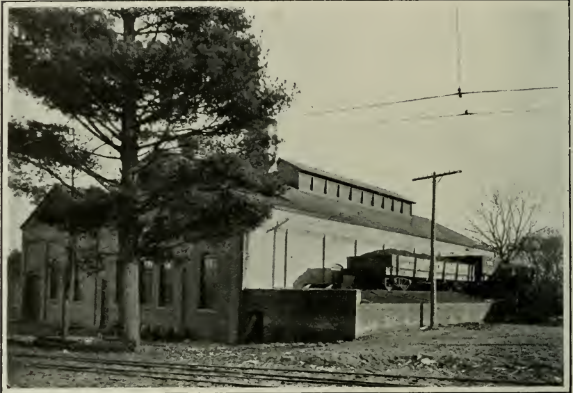
The track is standard gauge, laid with 70-pound T-rails, and is ballasted with coarse gravel and drained by vitrified tiling. The power
