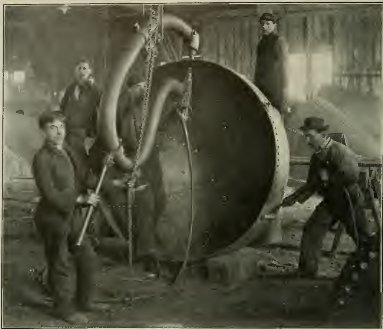
RIVETING UP BUOYS WITH PORTABLE TYPE PNEUMATIC RIVETER. Philadelphia Pneumatic Tool Company.
