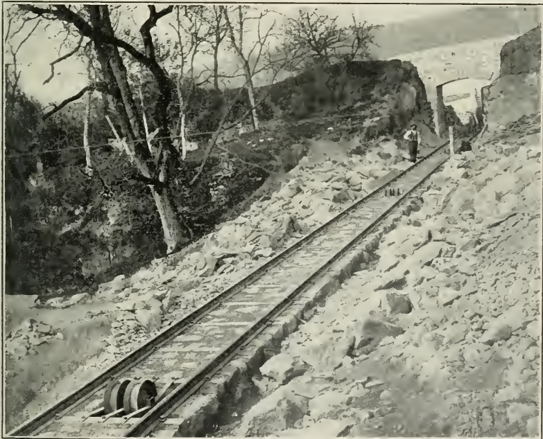
A PORTION OF THE COMPLETED PERMANENT WAY.
