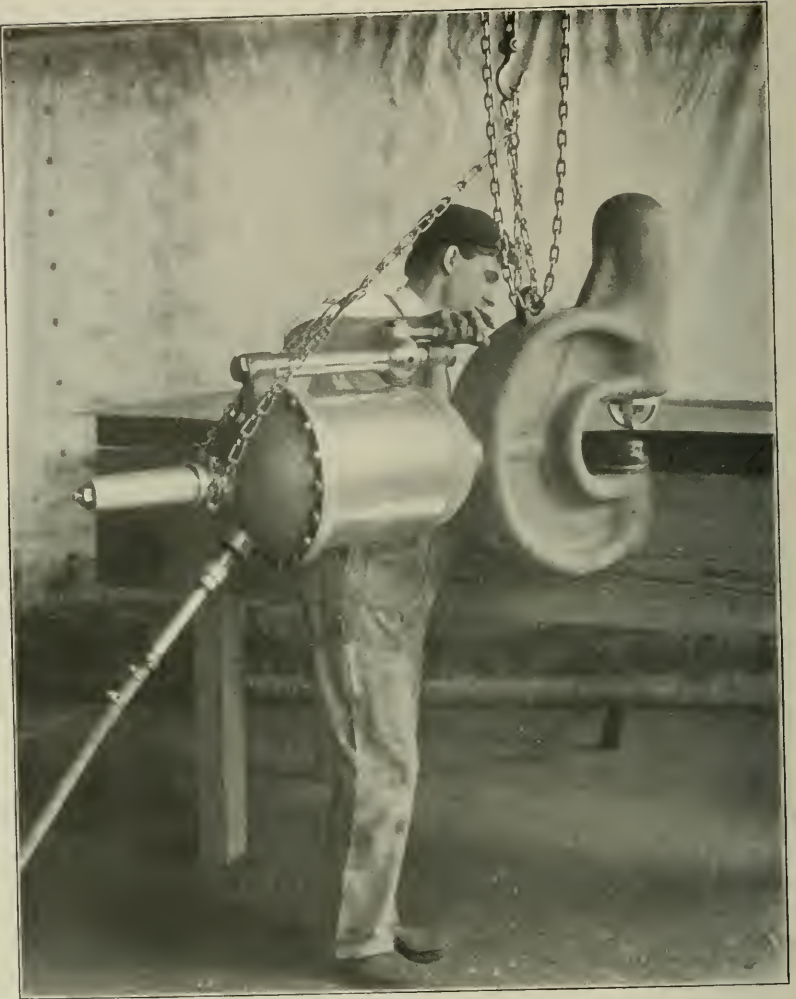
CASKEY PNEUMATIC PUNCH IN OPERATION.
