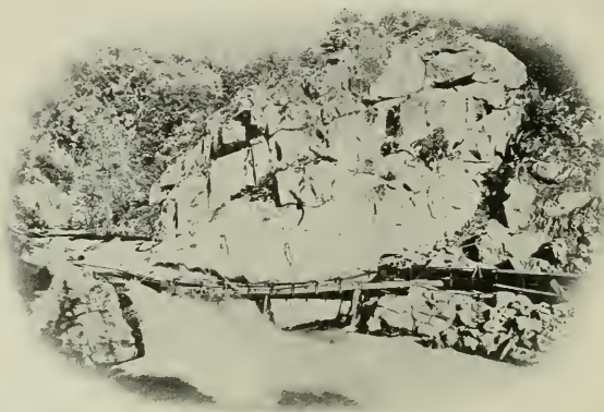
LUMBER CHUTE, FLUME, AND TRESTLE, MT. WHITNEY POWER CO.
