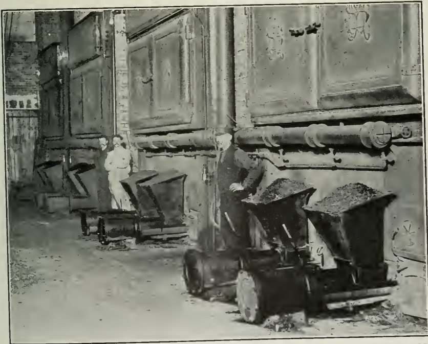
INSTALLATION OF UNDERFEED STOKERS IN DEPARTMENT STORE OF MARSHALL FIELD & CO., CHICAGO. The Underfeed Stoker Co. of America, Chicago, Ill.
