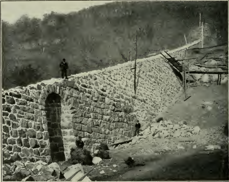
THE SUBSTRUCTURE OF THE VEVEY-MONT PÉLERIN RAILWAY.
