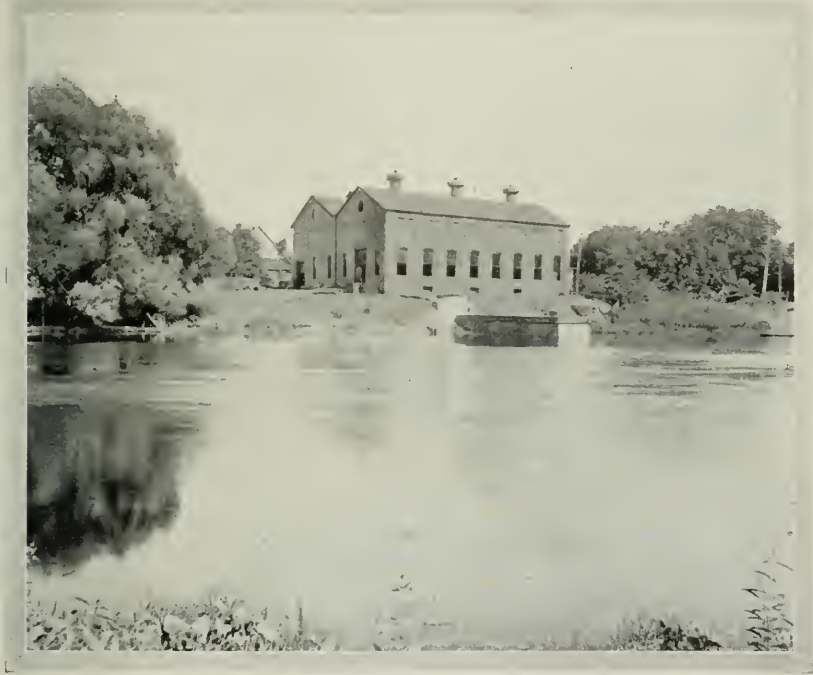
EXTERIOR OF POWER HOUSE, DETROIT, YPSILANTI & ANN ARBOR RAILWAY, YPSILANTI, MICH.
