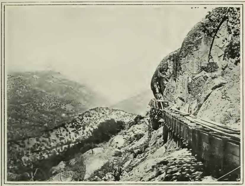
THE FLUME OF THE MT. WHITNEY POWER PLANT.
