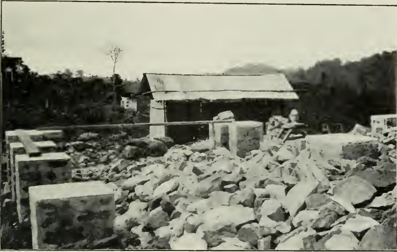
FOUNDATIONS FOR A TRADING STORE, GOLD-COAST AMALGAMATED MINES, ADJA BIPPO.
