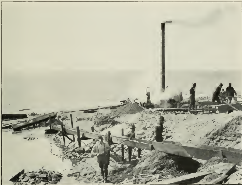
SLUICING ON THE BEACH NEAR NOME CITY.
