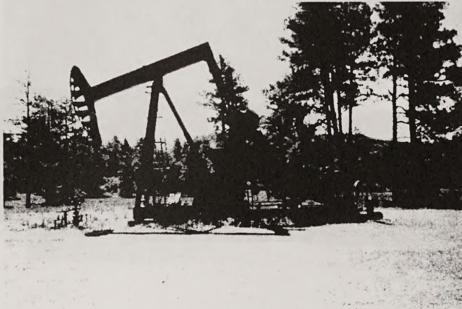
Photo 3-12 Typical CBM Well Facilities - Immediate Foreground View (0-300 feet)
