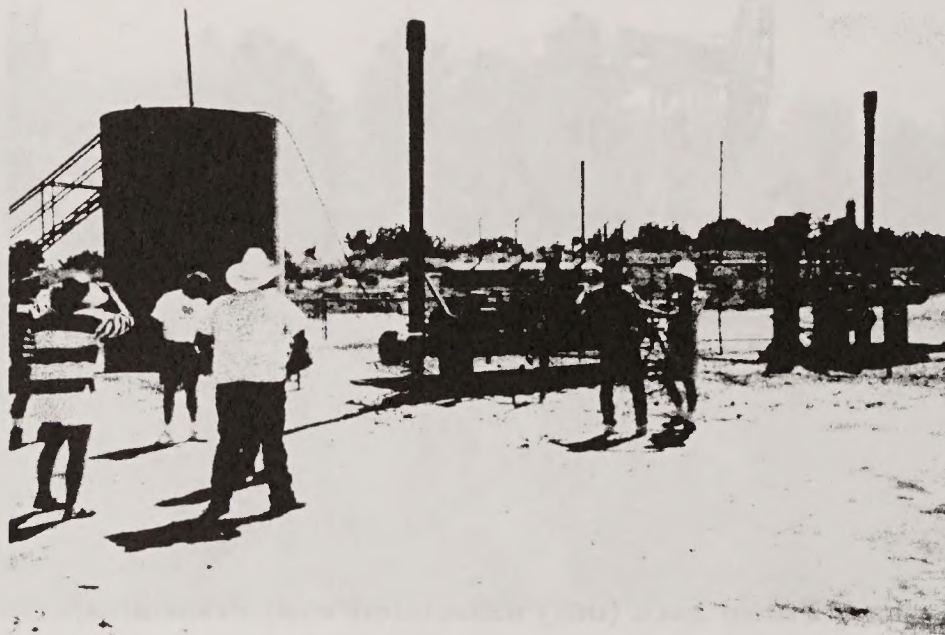
Photo 3-6 Typical Condensate Tank (only associated with conventional wells)
