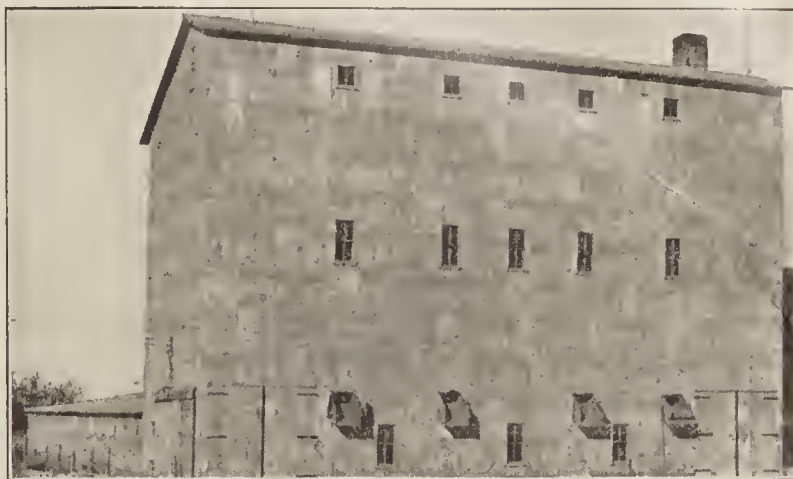
Funks New Corn Dryer, Warehouse and Elevator on the Funk Farms near Bloomington, Illinois
