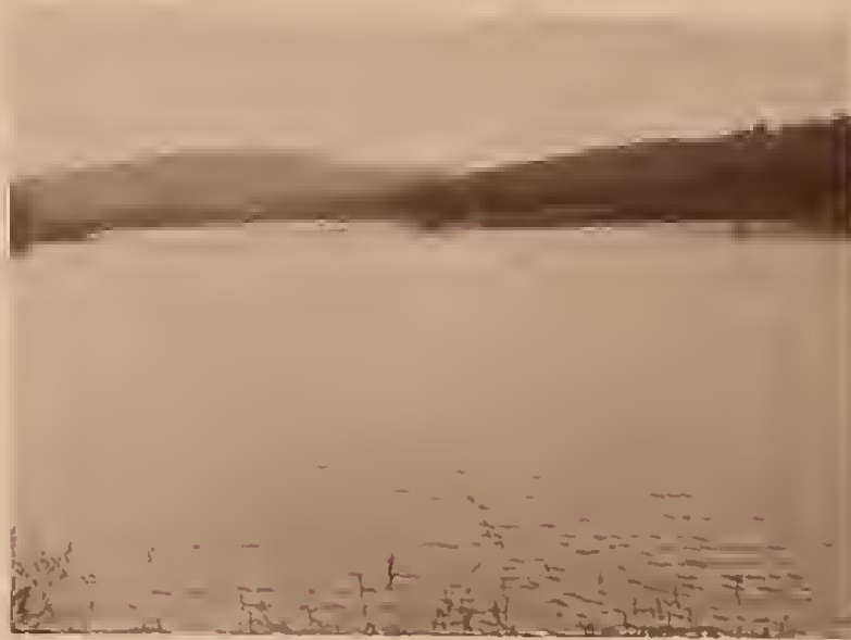
CV-1911 Atkins Reservoir
