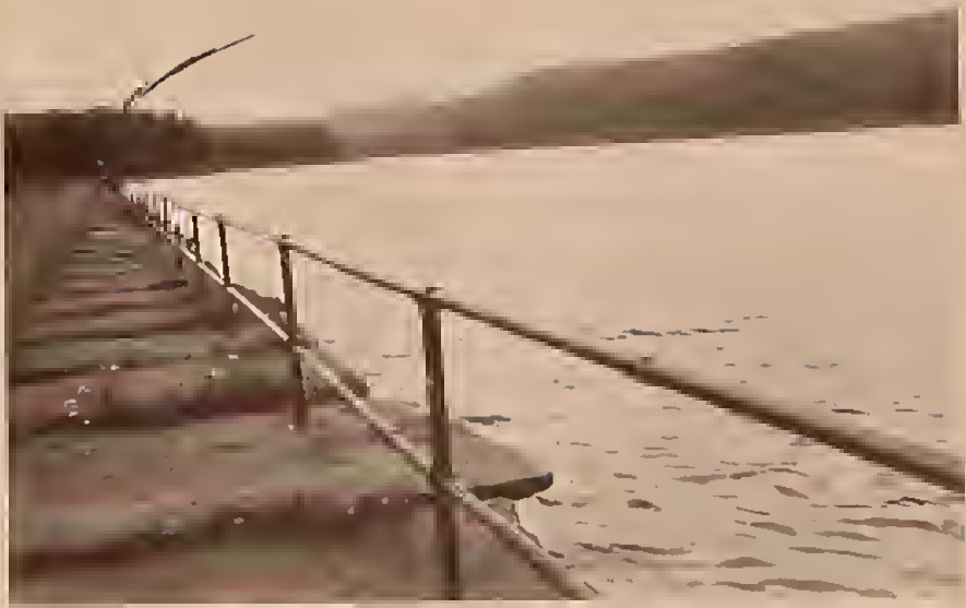
CV-2605 Whiting St. Reservoir
