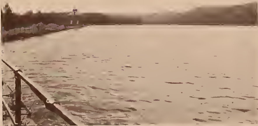
CV-2605 Whiting St. Reservoir
