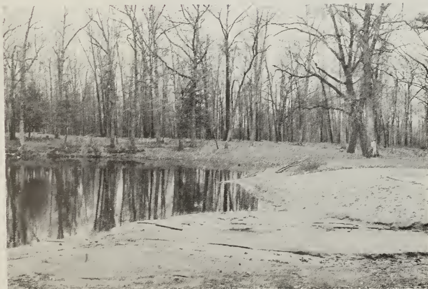
SC-4812 Turner Park Dam
