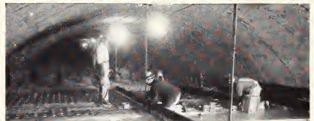
Above—Workmen shown laying the glass tile on a scaffolding; concrete will be poured over to comprise the ceiling. The tile, made by Sealed Joint Products Co., are held in place by Bronze grippers, shown at right, which are gripped by the concrete
