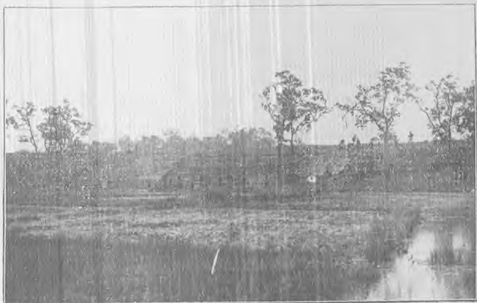
Dyke Repair Works, 1930.
