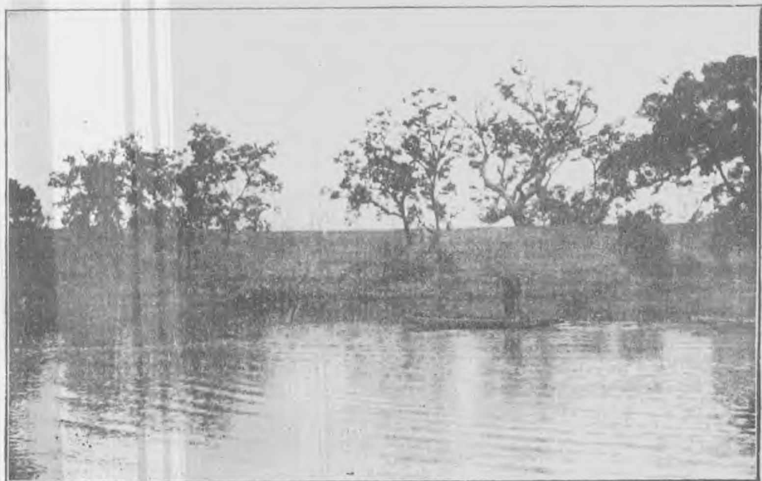
Dyke Repair Works, 1930.
