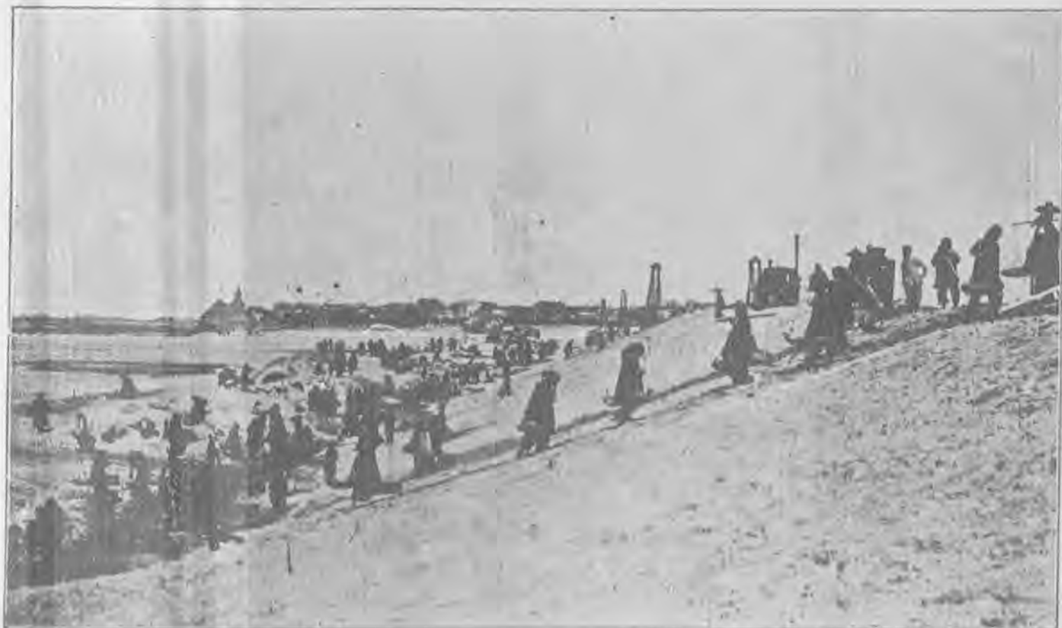
Lupao Control Sluice.
