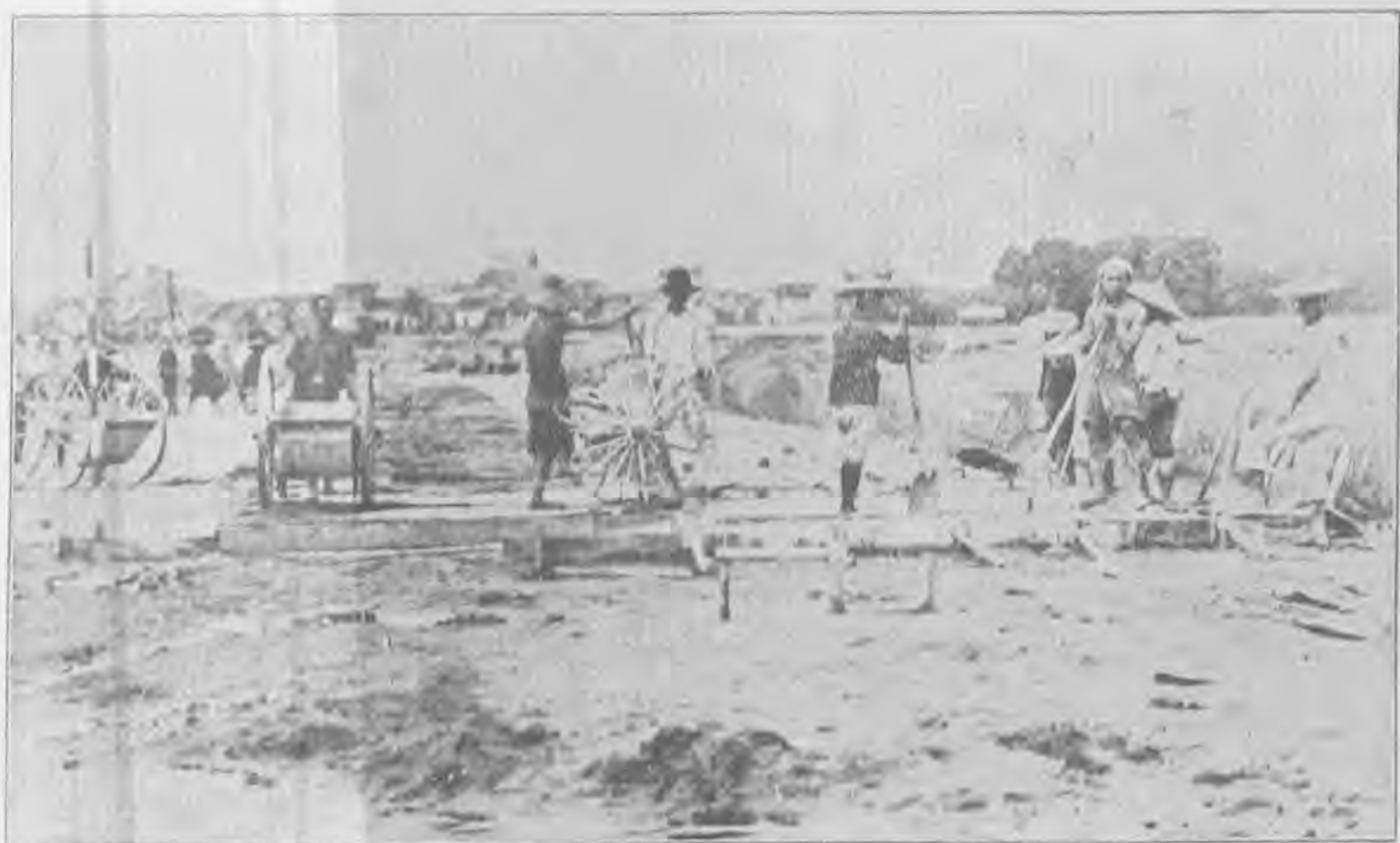
Lupao Control Sluice. Construction of flexible concrete-jacket on downstream apron.
