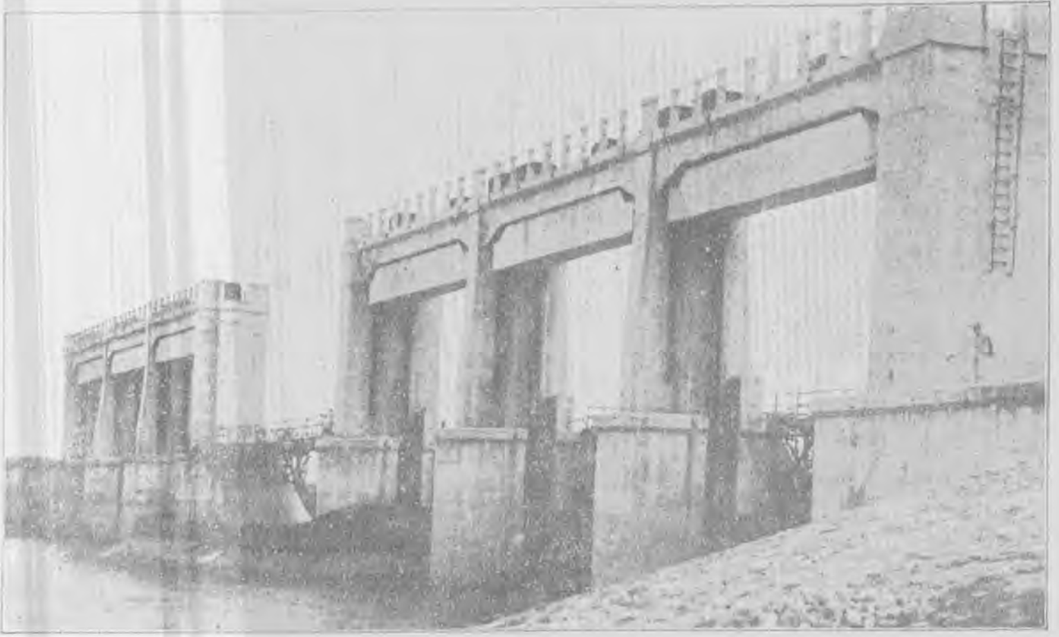
Lupao Control Sluice.
