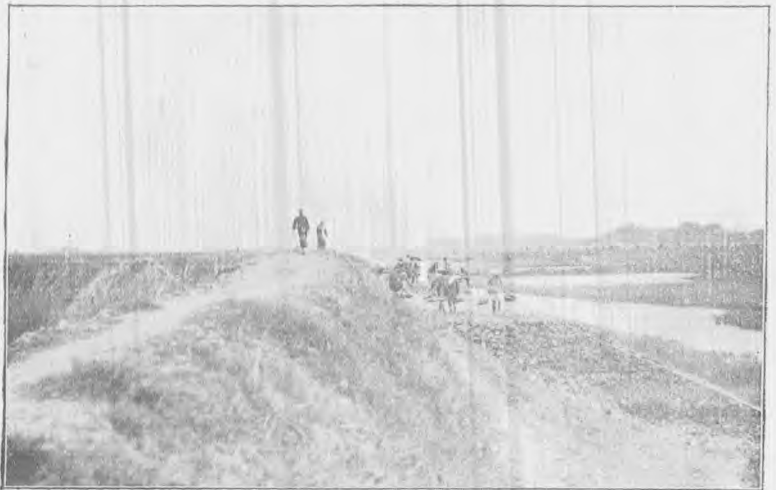
Dyke Repair Works, 1930.
