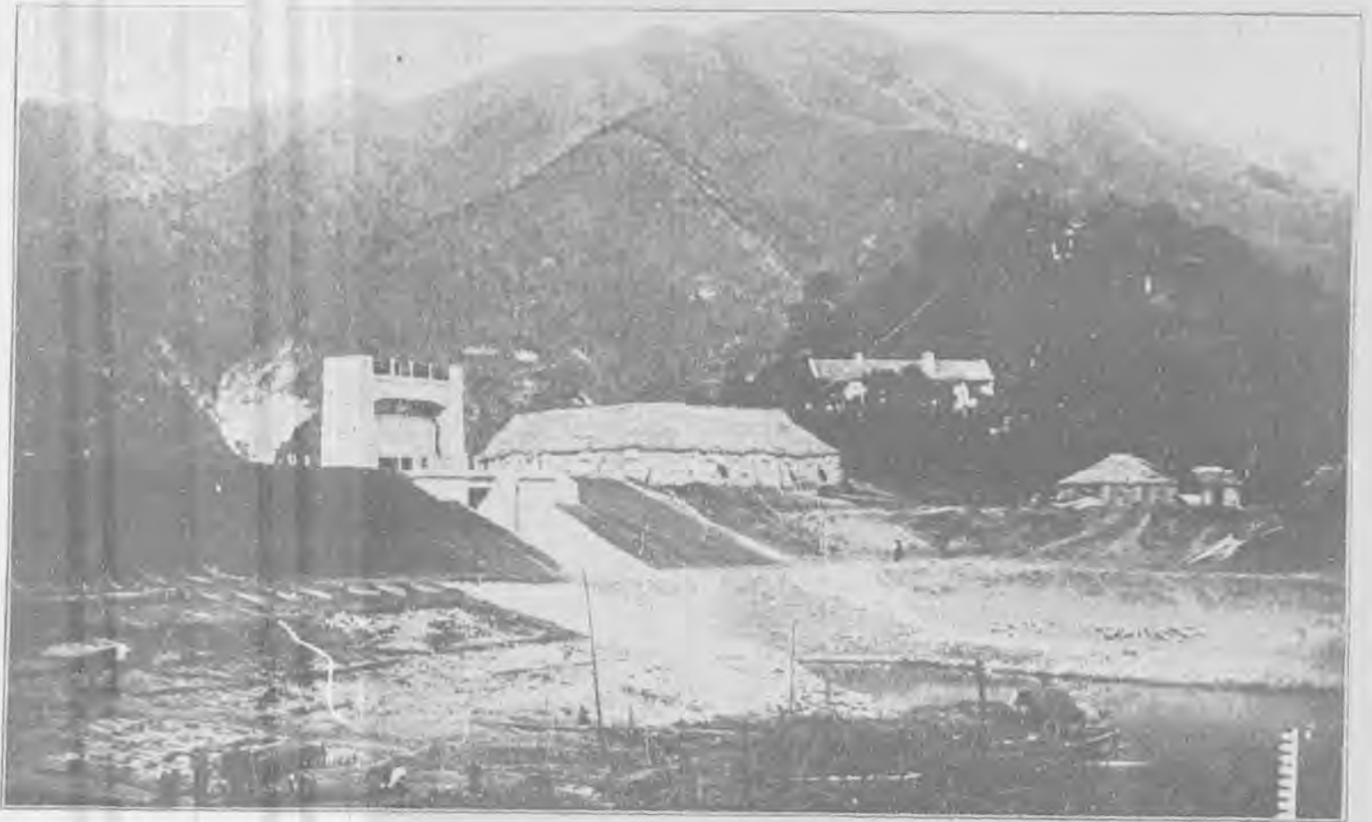
Sunglung Control Sluice.
