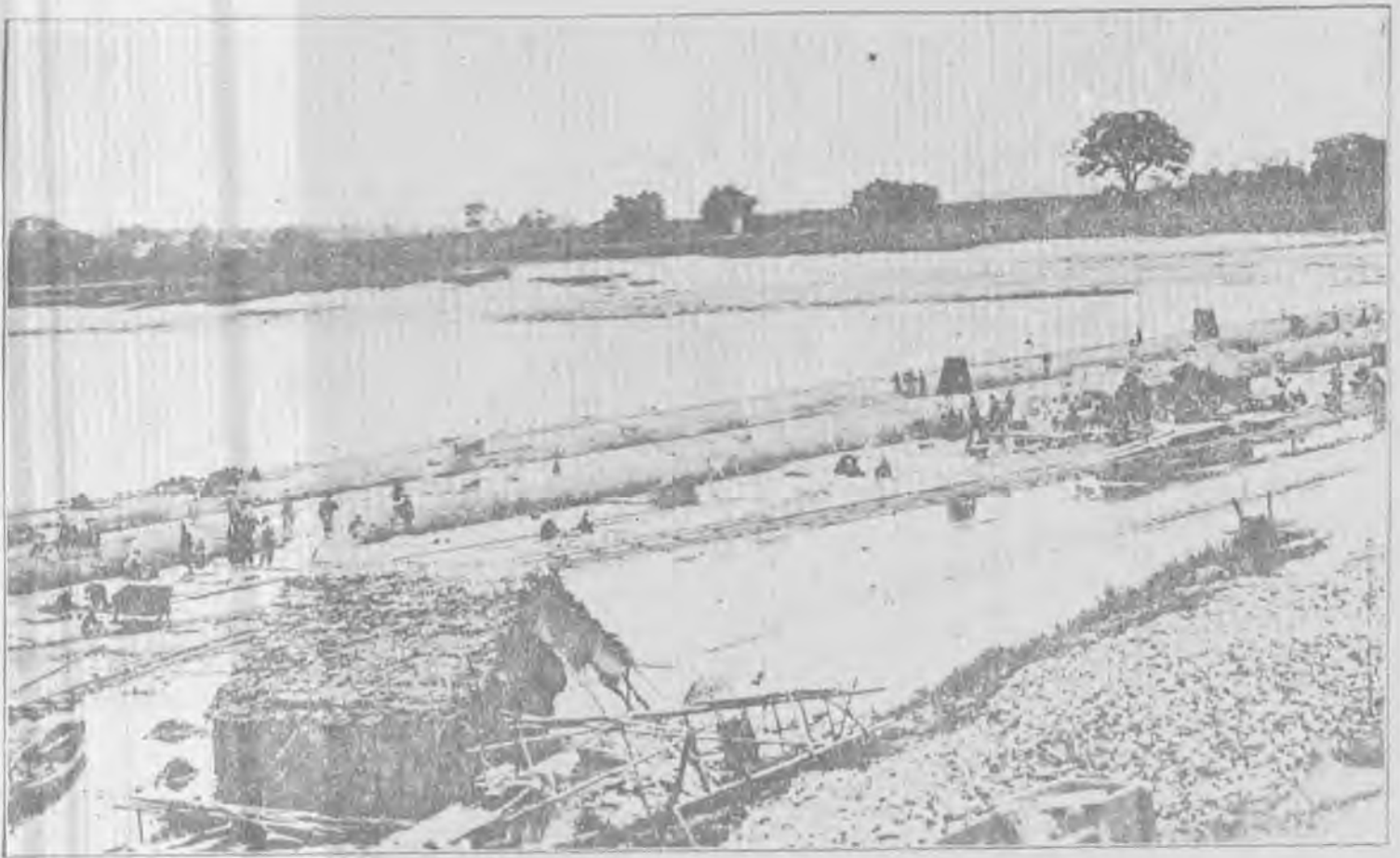
Lupao Control Sluice.
