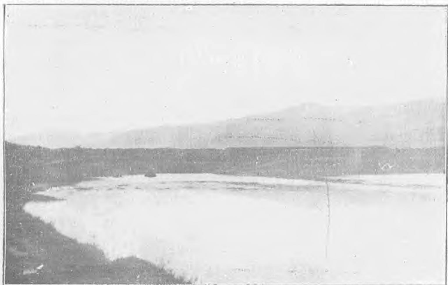
Newly refilled wash-out at Tung Chuen Dyke. (1930)
