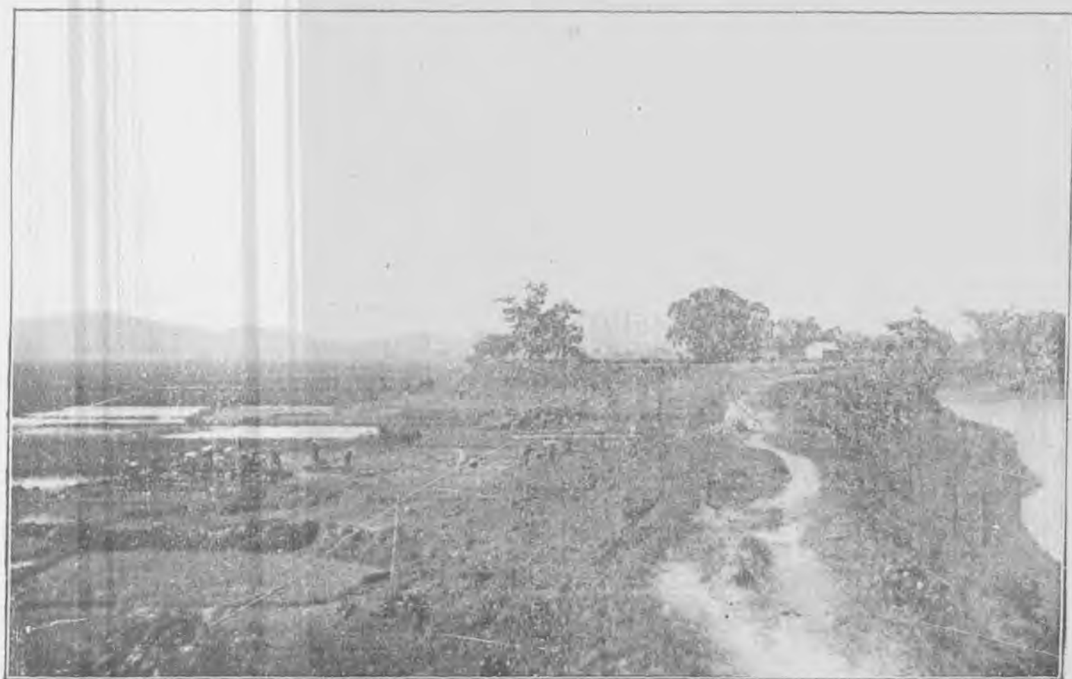
Dyke Repair Works, 1930.
