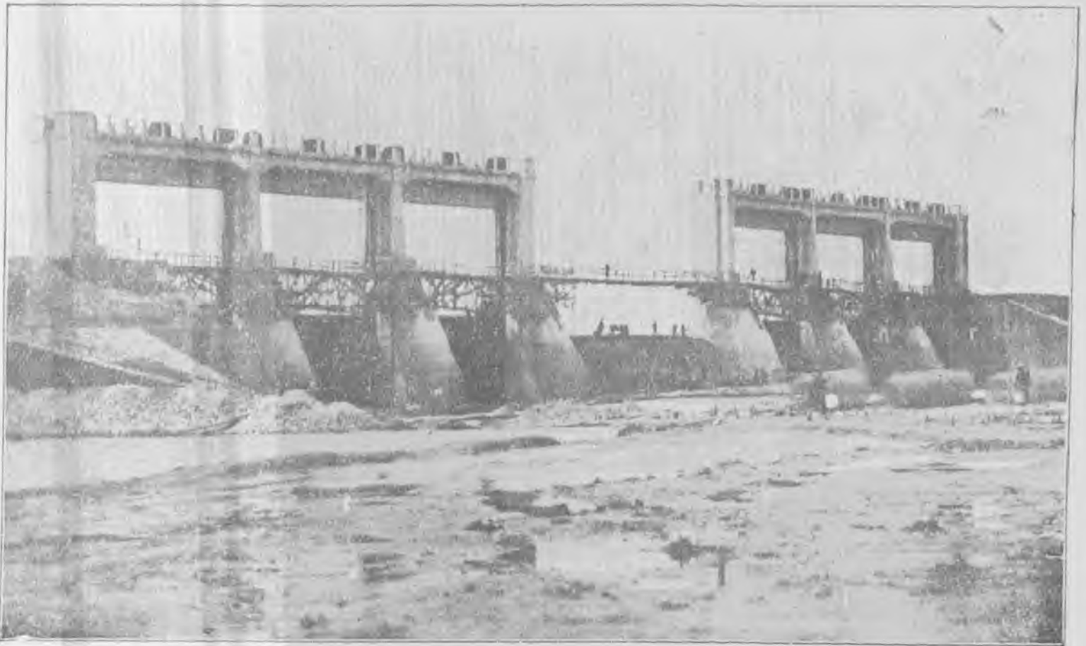
Lupao Control Sluice.
