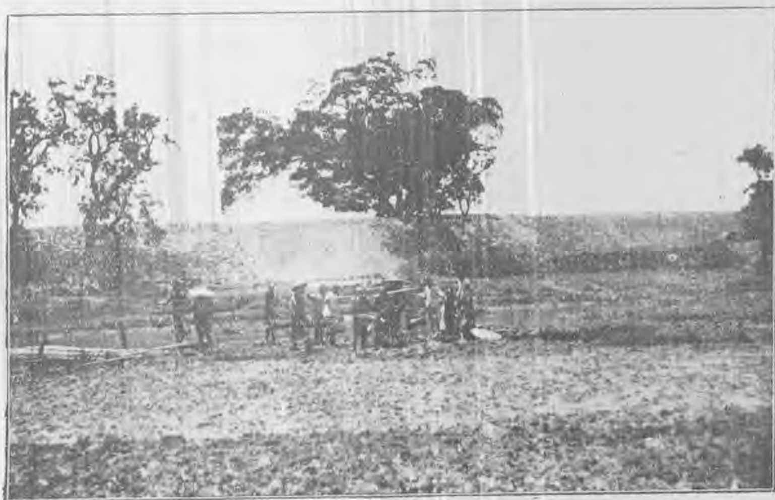
Dyke Repair Works, 1930.
