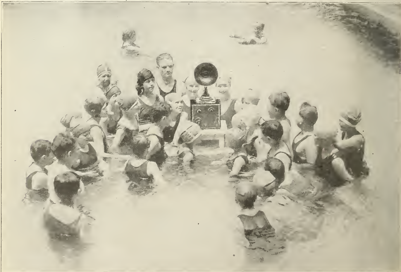
RADIO INSTALLED IN SOCIETY SWIMMING POOL
