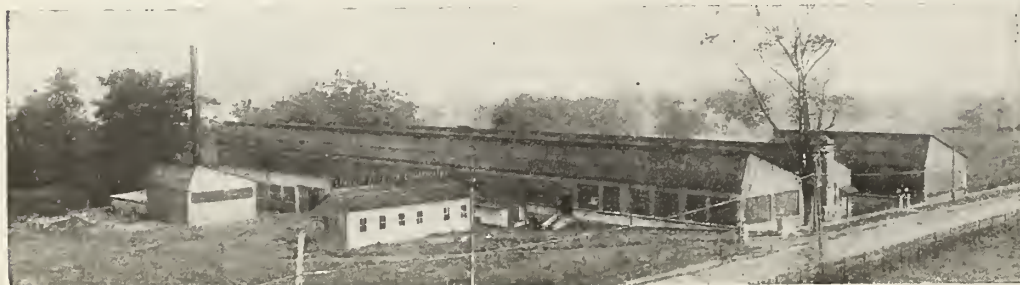
The New Liberty Electric Corp. Factory at Stamford, Conn.
