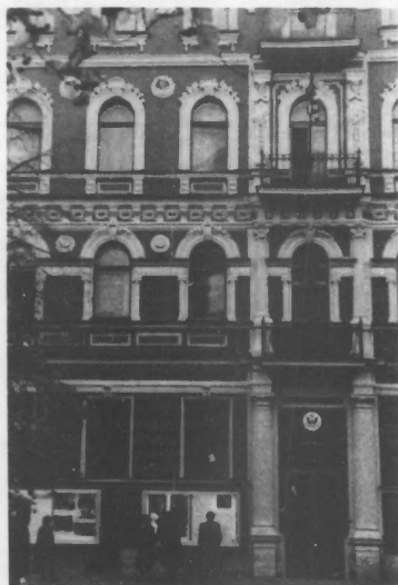
LENINGRAD, USSR—New front of the U.S. consulate general here, after restorative work had been completed.
