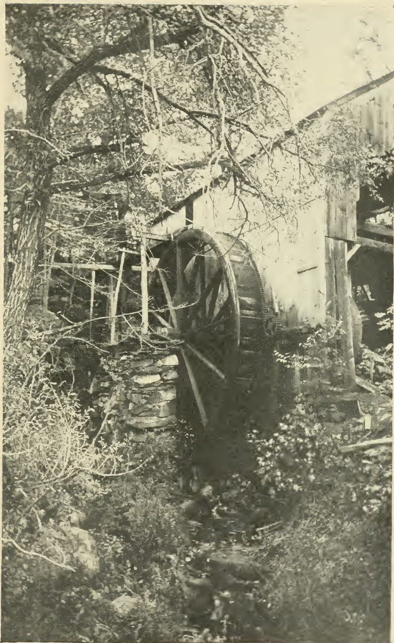
Mill at Merwinsville on the Housatonic.
