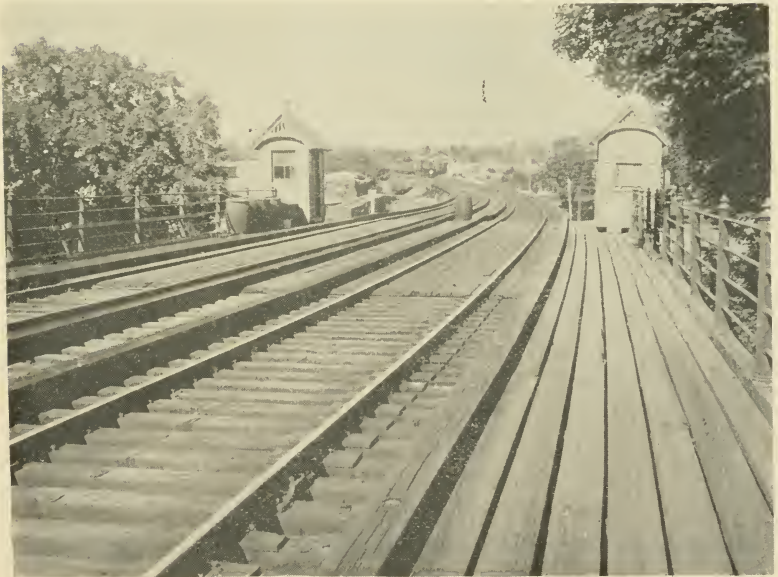
Approach of the Poughkeepsie Bridge.
