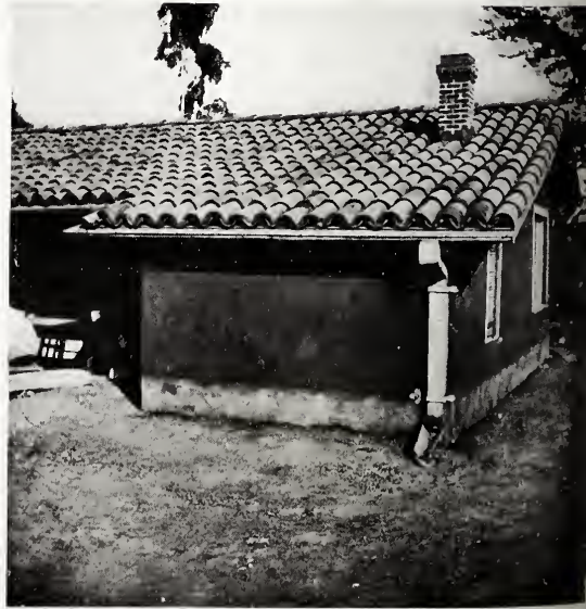
AN OLD MISSION TILED ROOF LEFT TO THE DESTRUCTION OF TIME. THE OLD TILES ARE ILL AT EASE NEAR A SMOOTH MODERN ROOF. SHOWING THE IRREGULARITY OF THE OLD HAND-MADE TILES.
