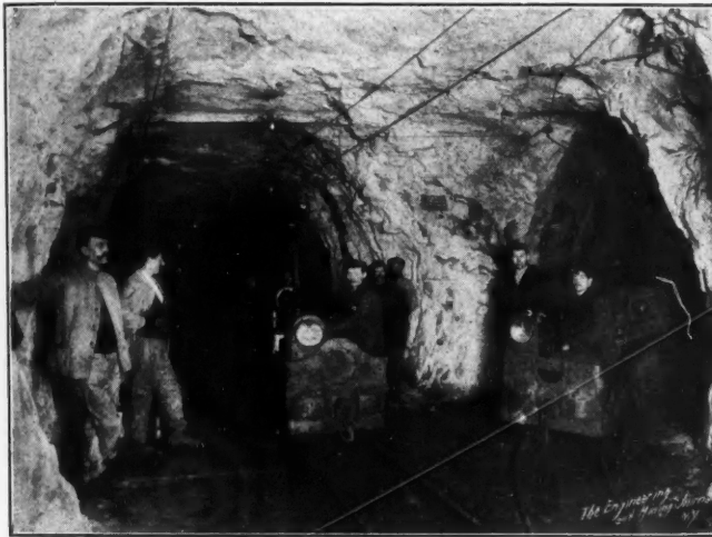
UNDERGROUND ELECTRIC HAULAGE IN THE BRIEY DISTRICT
